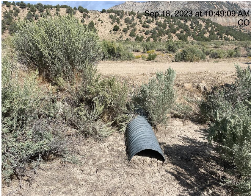
Photo # 9566 Culvert needs maintenance
