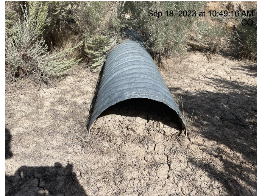
Photo # 9567 Culvert needs maintenance
