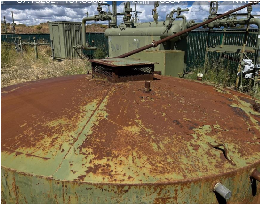
Photo #1. View of corrective action identified in FIR Doc.#712700638.
