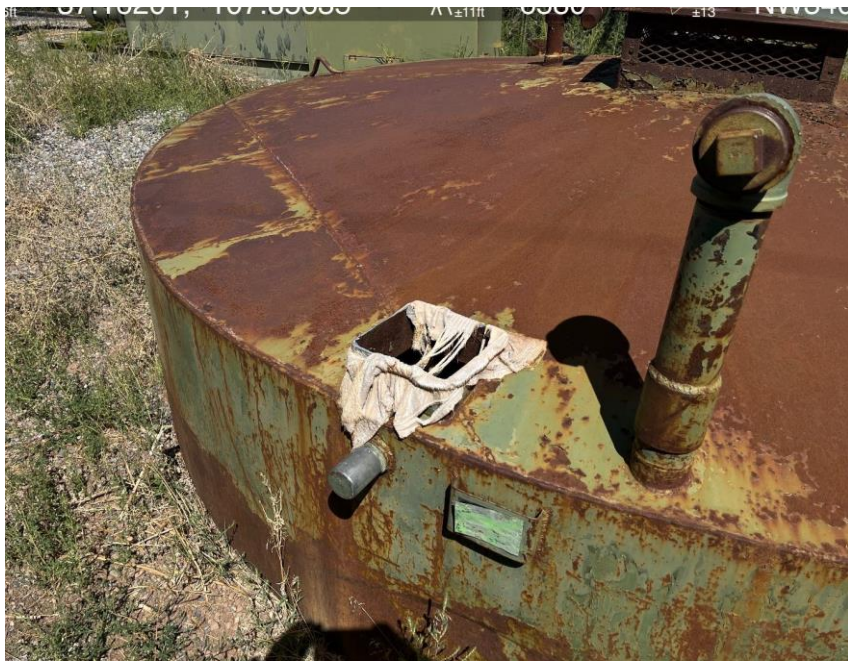
Photo #3. View of corrective action identified in FIR Doc.#712700638.
