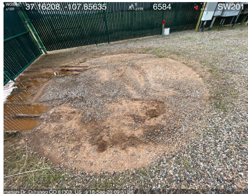
Photo #4. View of removed tank, resolved corrective action.
