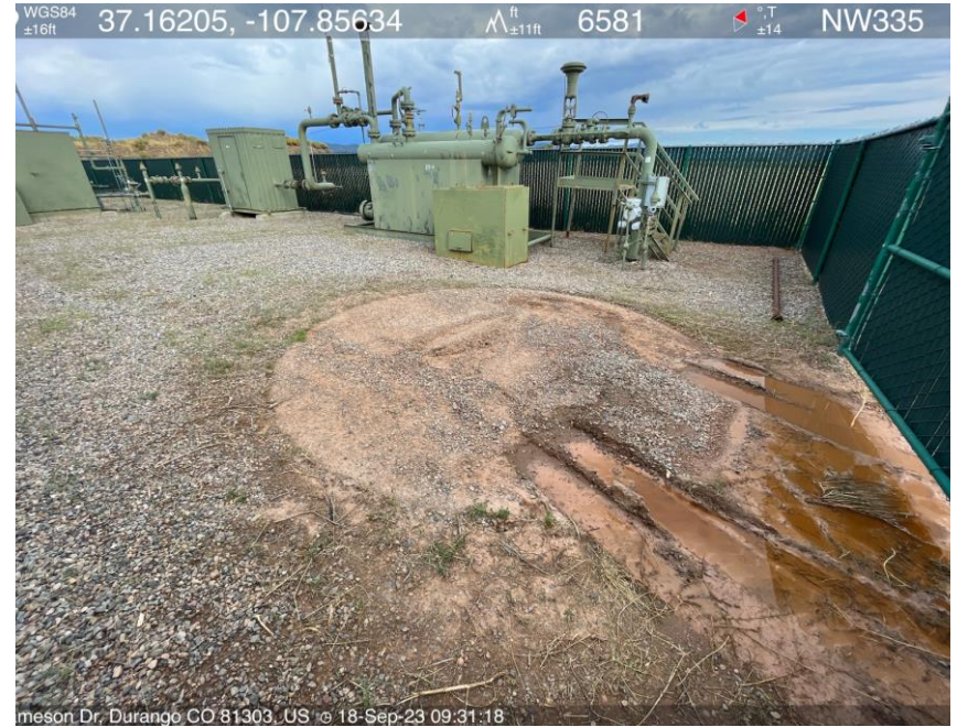
Photo #2. View of removed tank, resolved corrective action.
