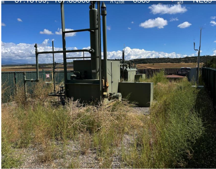
Photo #1. View of corrective action identified in FIR Doc.#712700639.
