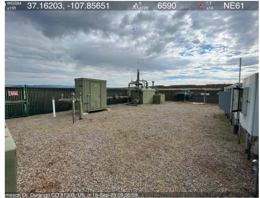
Photo 2. View of completed corrective action.
