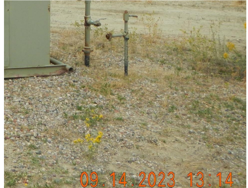
Open end unused 1" flowline at separators
