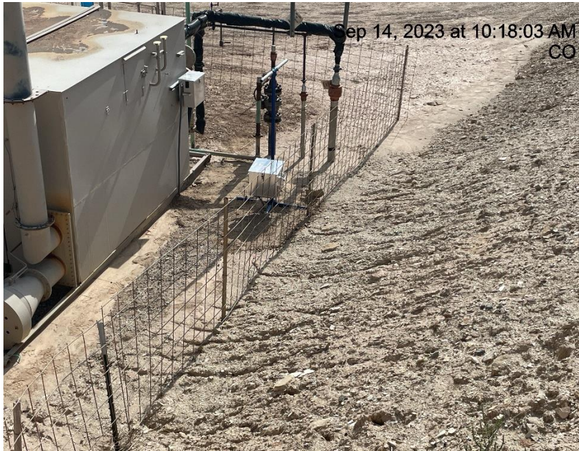
Photo # 9296 Erosion on slope & transport of sediment onto location/insufficient BMP's
