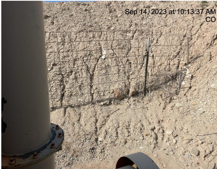
Photo # 9282 Erosion on slope & transport of sediment onto location/insufficient BMP's
