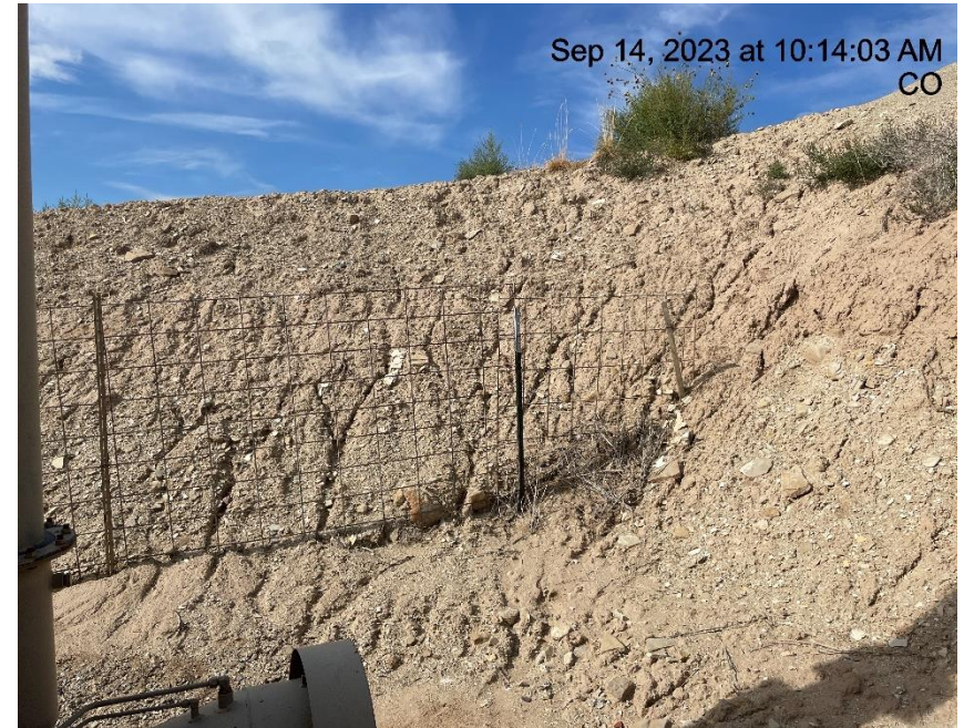
Photo # 9286 Erosion on slope & transport of sediment onto location/insufficient BMP's
