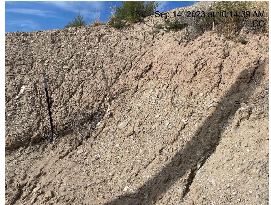
Photo # 9290 Erosion on slope & transport of sediment onto location/insufficient BMP's
