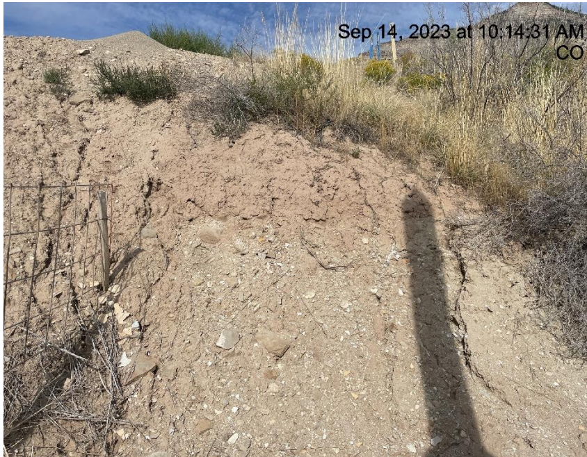
Photo # 9289 Erosion on slope & transport of sediment onto location/insufficient BMP's
