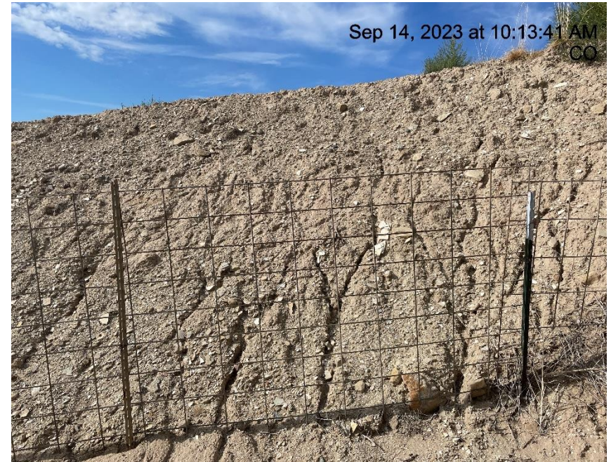
Photo # 9283 Erosion on slope & transport of sediment onto location/insufficient BMP's
