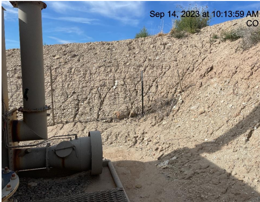
Photo # 9285 Erosion on slope & transport of sediment onto location/insufficient BMP's
