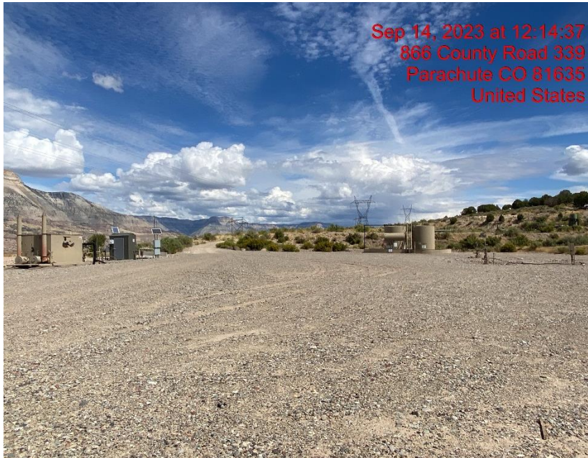
West End of Location – Photo #06406
