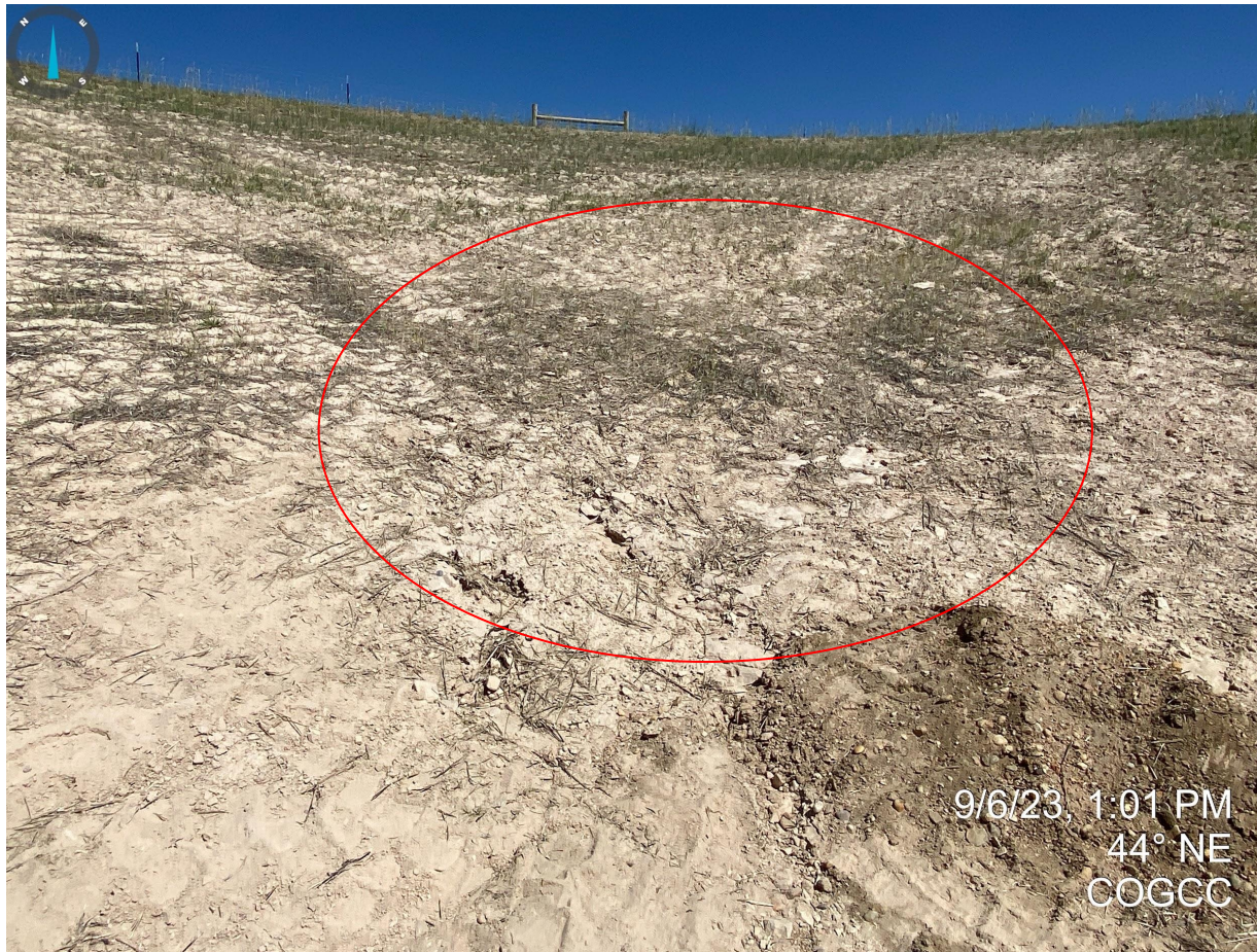
Photo 6. Taken from the northeast corner of the location. Photo illustrates that cut slopes do not appear to be properly stabilized as evidence by bare/exposed soils and no apparent stormwater controls to prevent erosion degradation (e.g. rilling).
