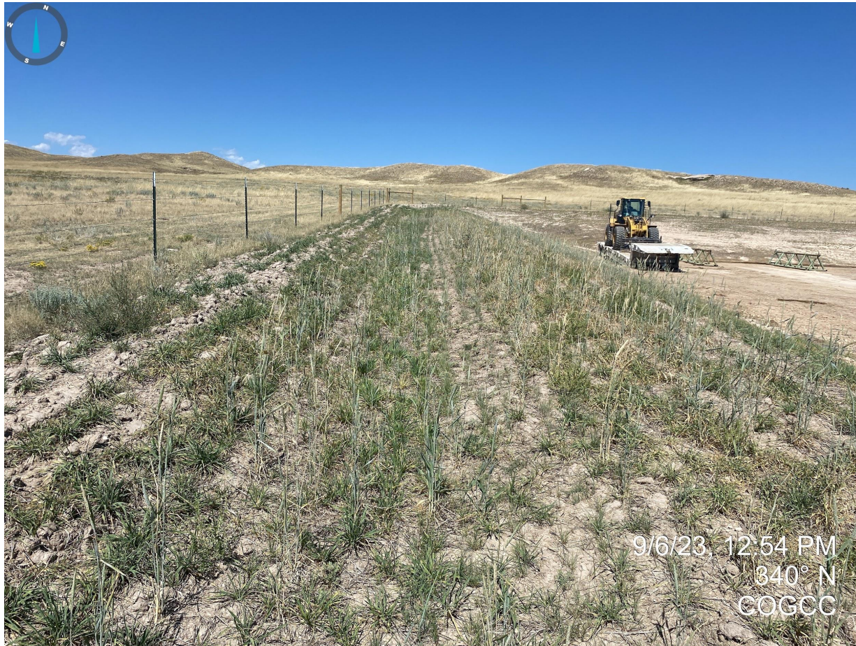
Photo 2. Taken near the locations entrance. It appears the Operator planted an annual crop species (e.g. triticale) as part of temporary stabilization. The Operator shall ensure the location is stabilized for longer term by utilizing desirable perennial plant species reflective of adjacent reference areas.
