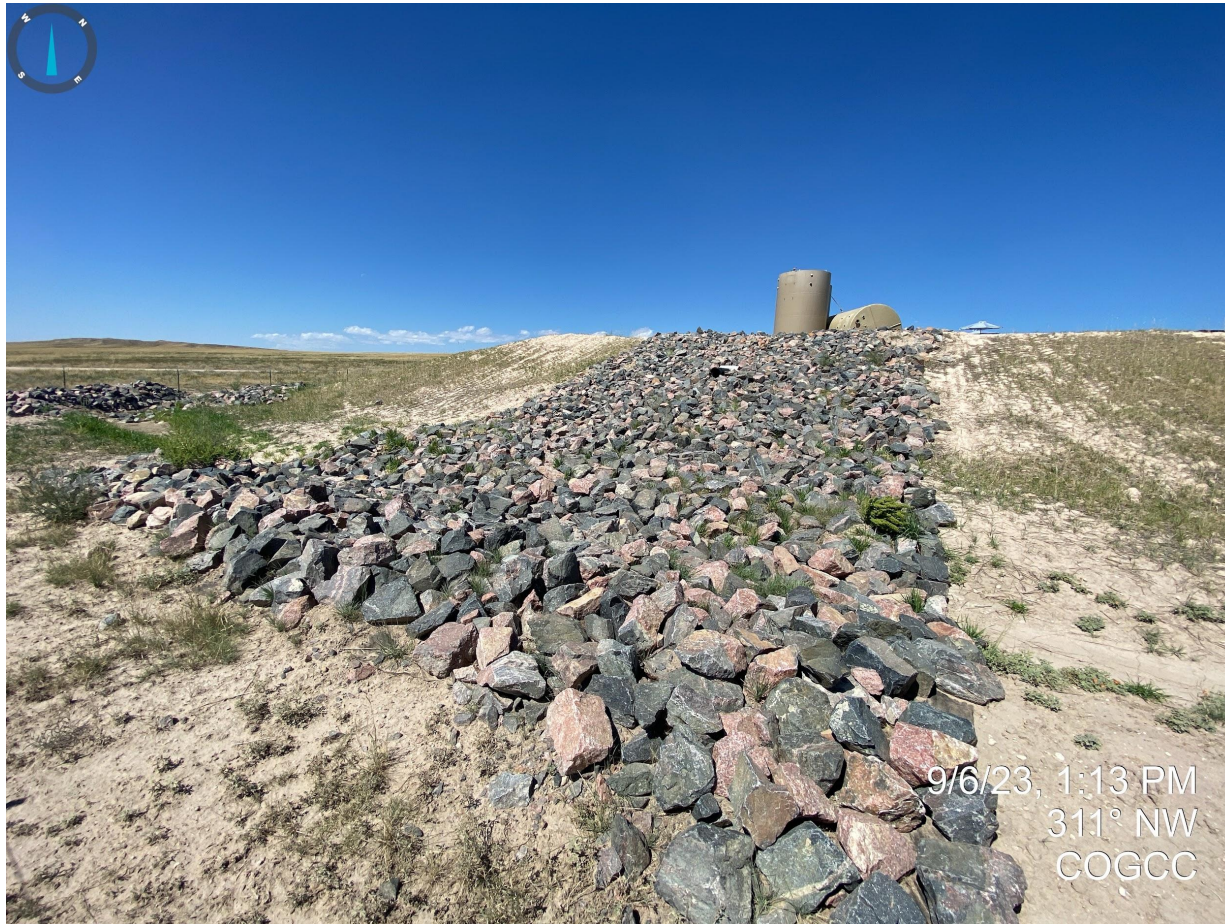
Photo 21. Taken from the southwest corner of the location. Photo illustrates armored outflow of sediment basin.
