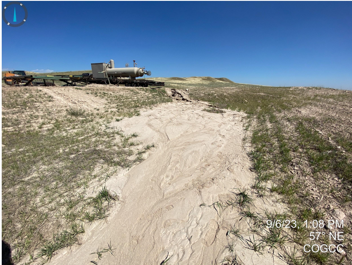
Photo 15. Taken within the southern sediment basin. Photo illustrates sediment deposition within the sediment trap. Maintenance and repairs are required in order to comply with Rule 1002.f.
