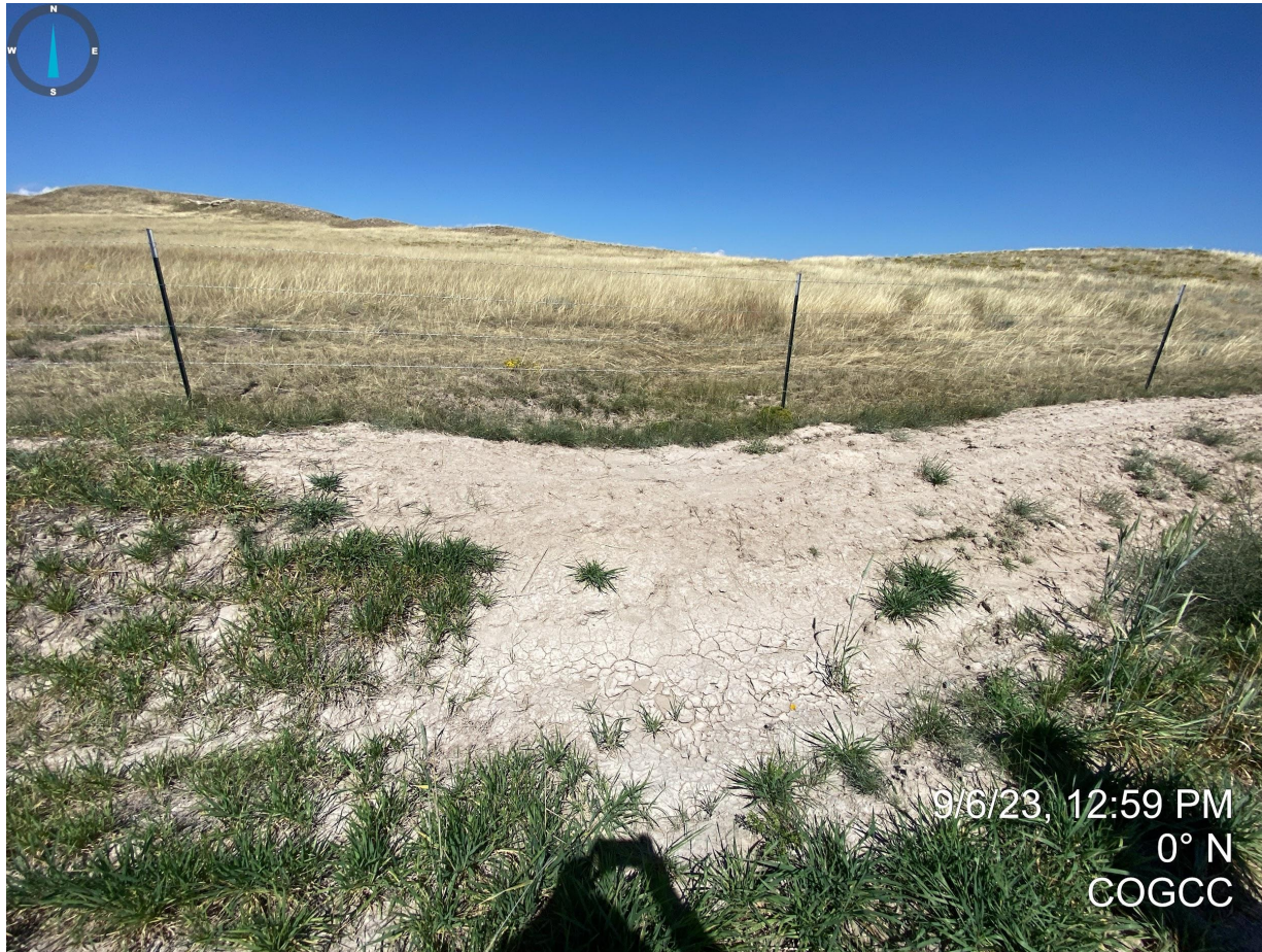
Photo 5. Taken from the center/northern portion of the location. Photo illustrates that the perimeter stormwater controls/BMPs do not appear to be adequate at controlling stormwater run on with evidence of sediment transport into the diversion ditch.
