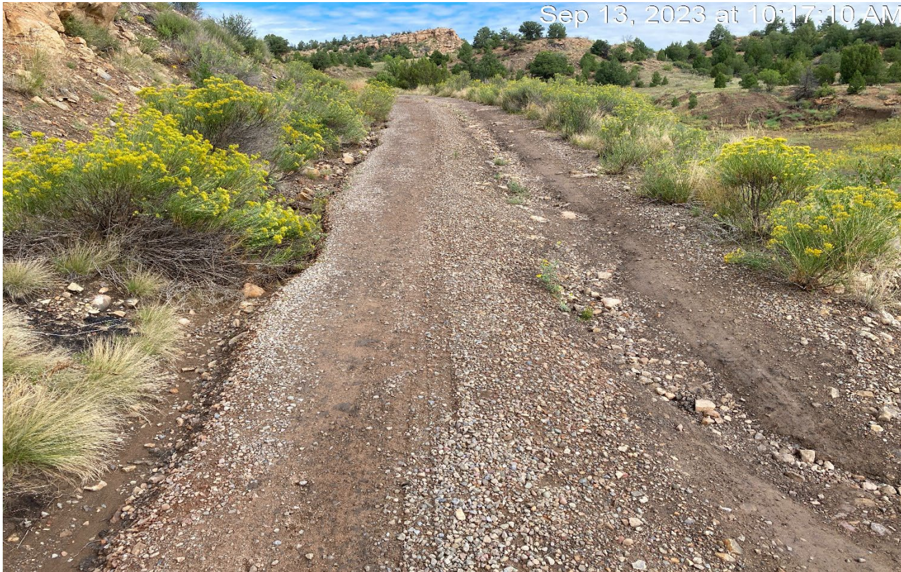
Photo 1. Facing north along the access road. There is erosion occurring along the road that needs to be repaired.
