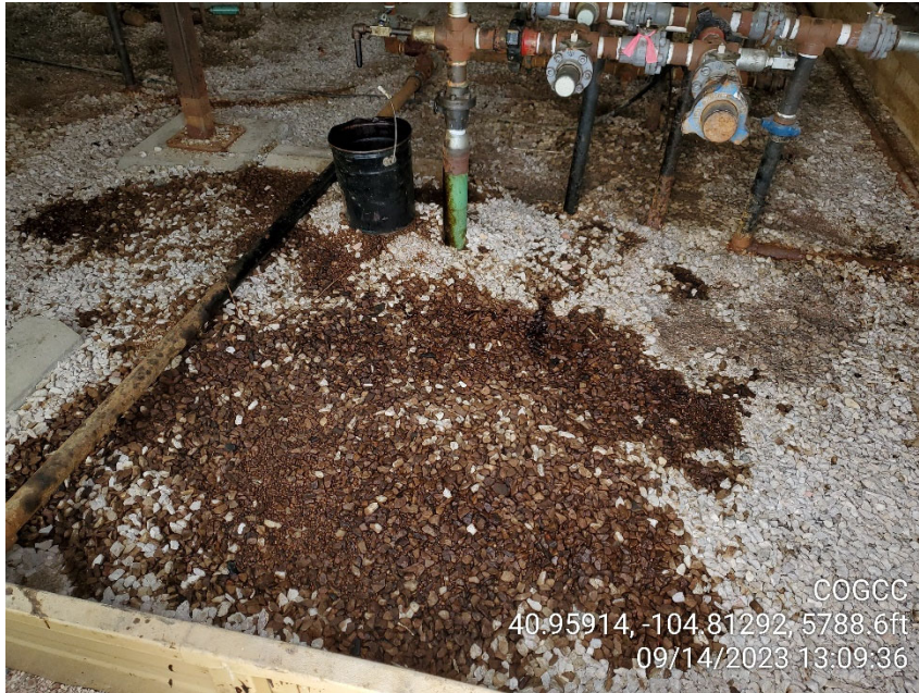
Photo 7 Evidence of blowdown onto ground in separator building
