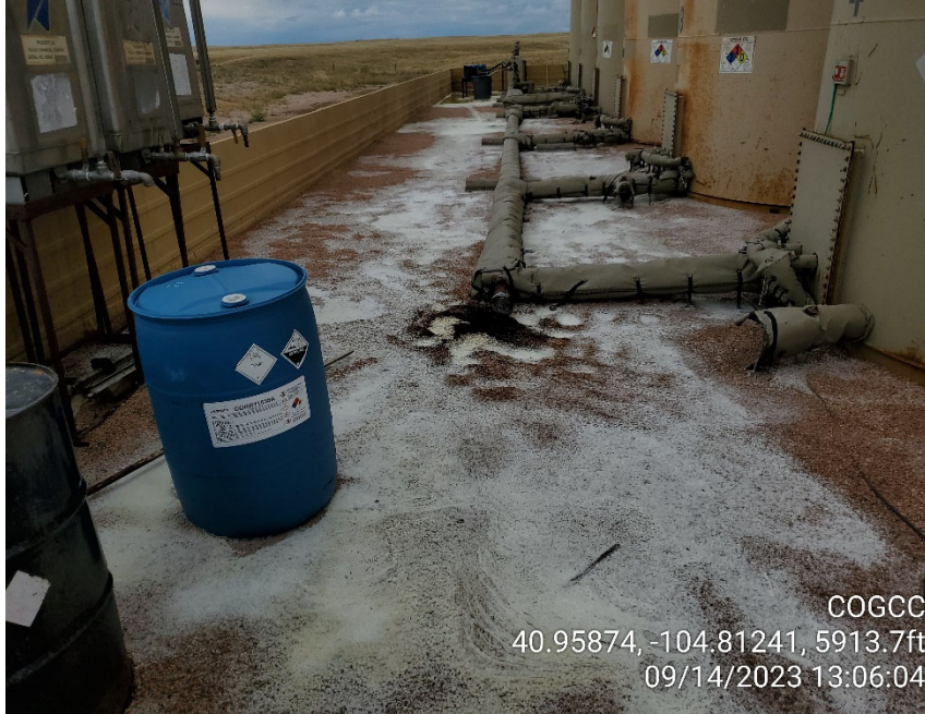
Photo 3 Salt crystals along south side of secondary containment
