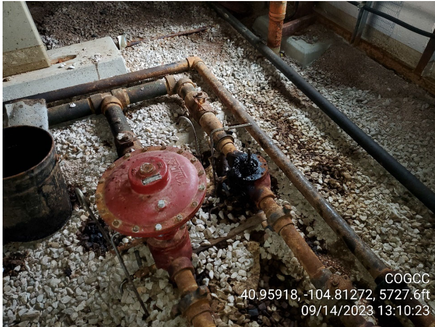
Photo 9 Leaking fittings inside separator building
