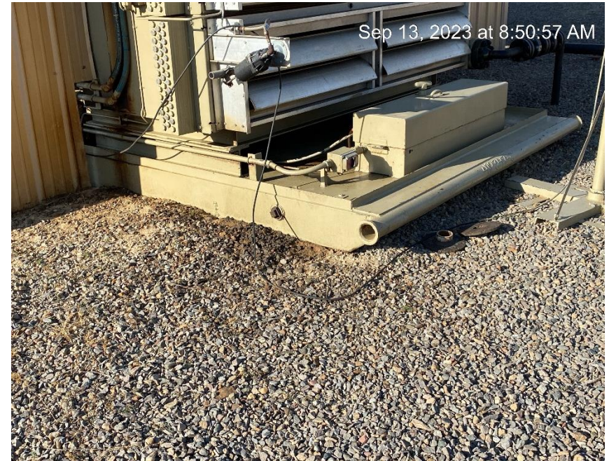
Staining around compressor
