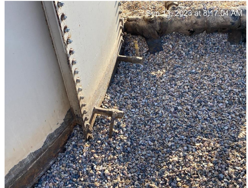
Open end tank valves
