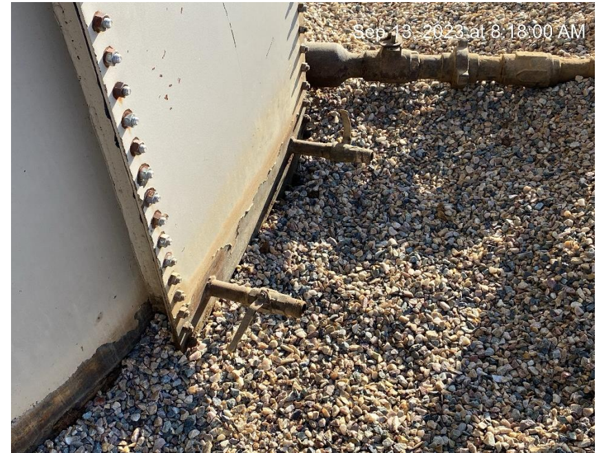
Open end tank valves
