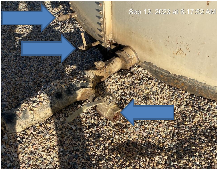
Open end tank valves
