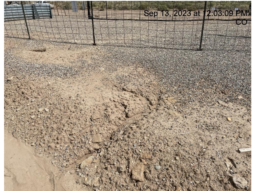
Photo # 9102 Erosion & transport of sediment/insufficient BMP's
