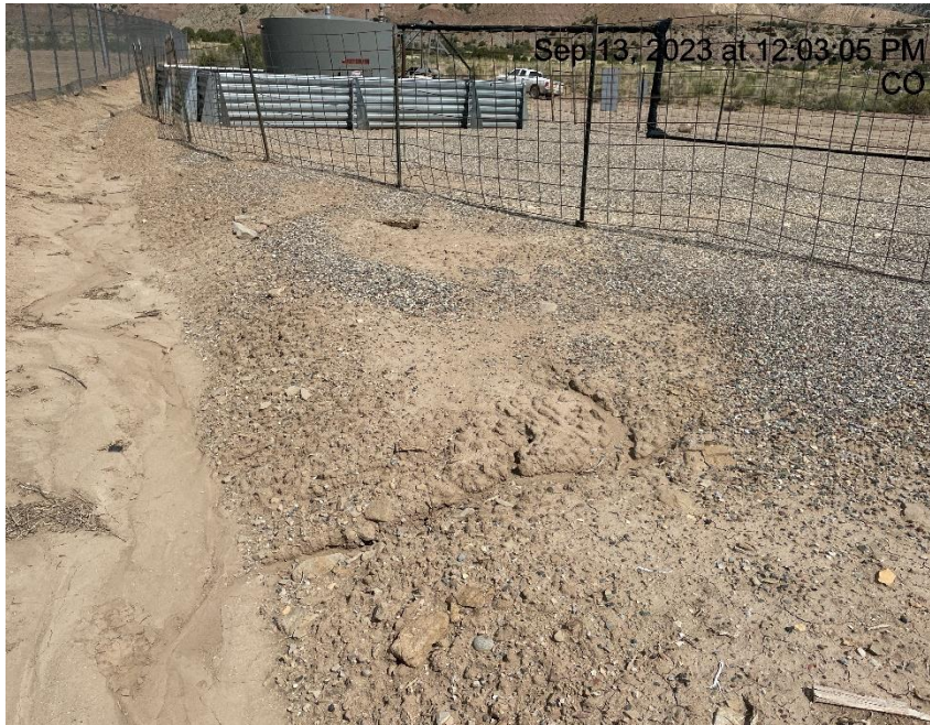
Photo # 9101 Erosion & transport of sediment/insufficient BMP's
