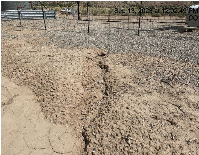
Photo # 9099 Erosion & transport of sediment/insufficient BMP's
