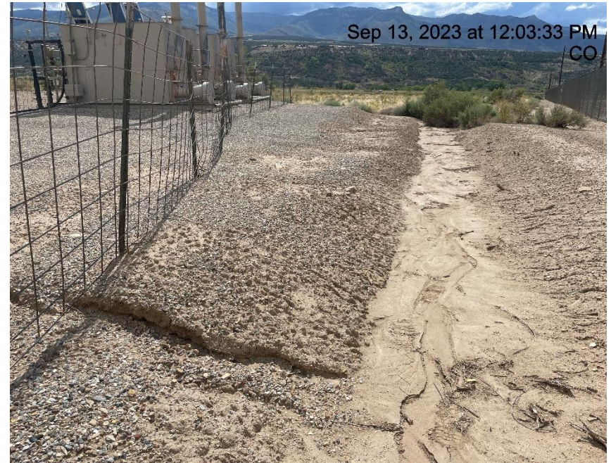
Photo # 9105 Erosion & transport of sediment/insufficient BMP's
