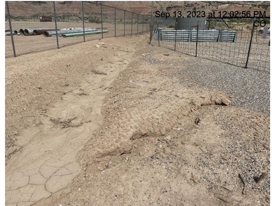
Photo # 9100 Erosion & transport of sediment/insufficient BMP's
