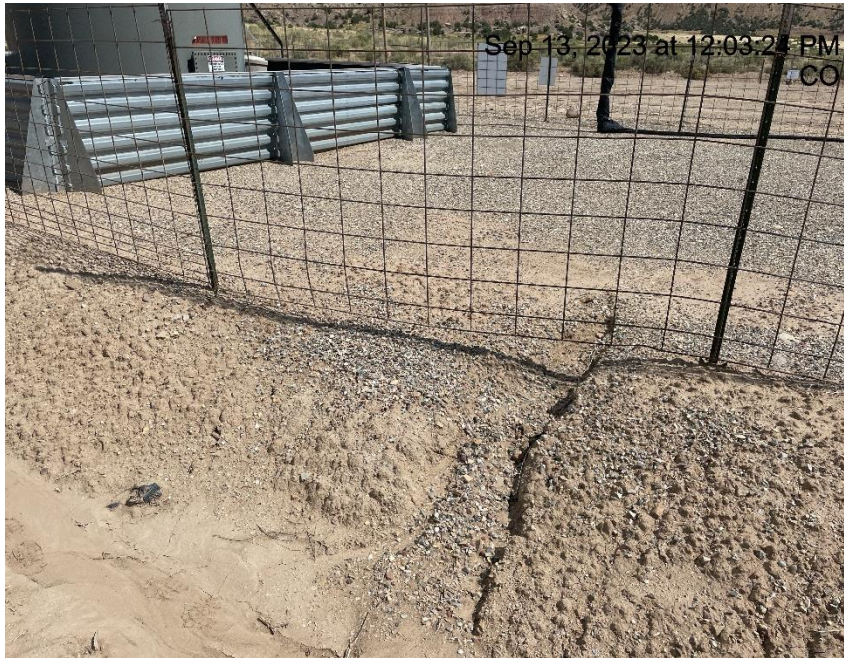
Photo # 9104 Erosion & transport of sediment/insufficient BMP's
