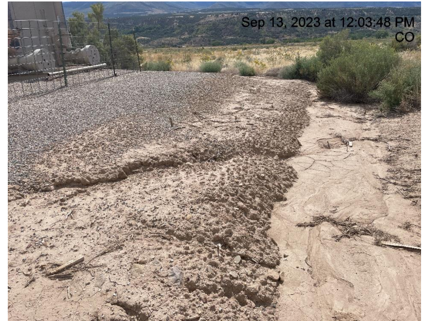
Photo # 9107 Erosion & transport of sediment/insufficient BMP's
