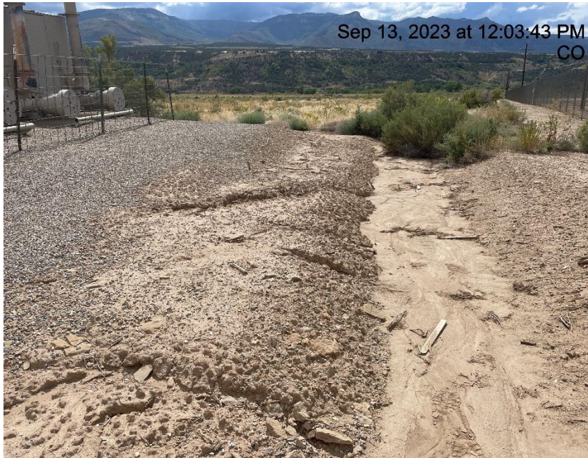
Photo # 9106 Erosion & transport of sediment/insufficient BMP's
