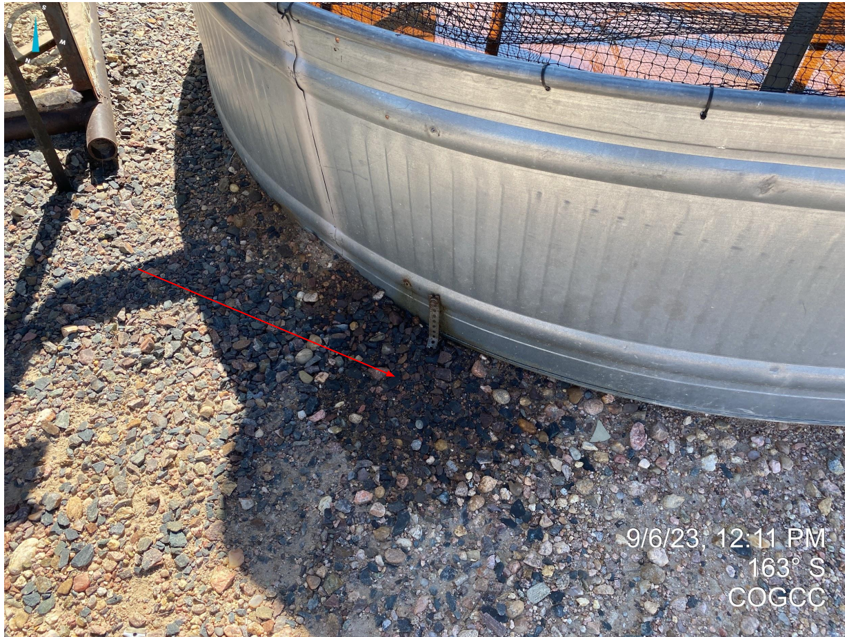
Photo 14. Stained soil at day tank next to compressor.
