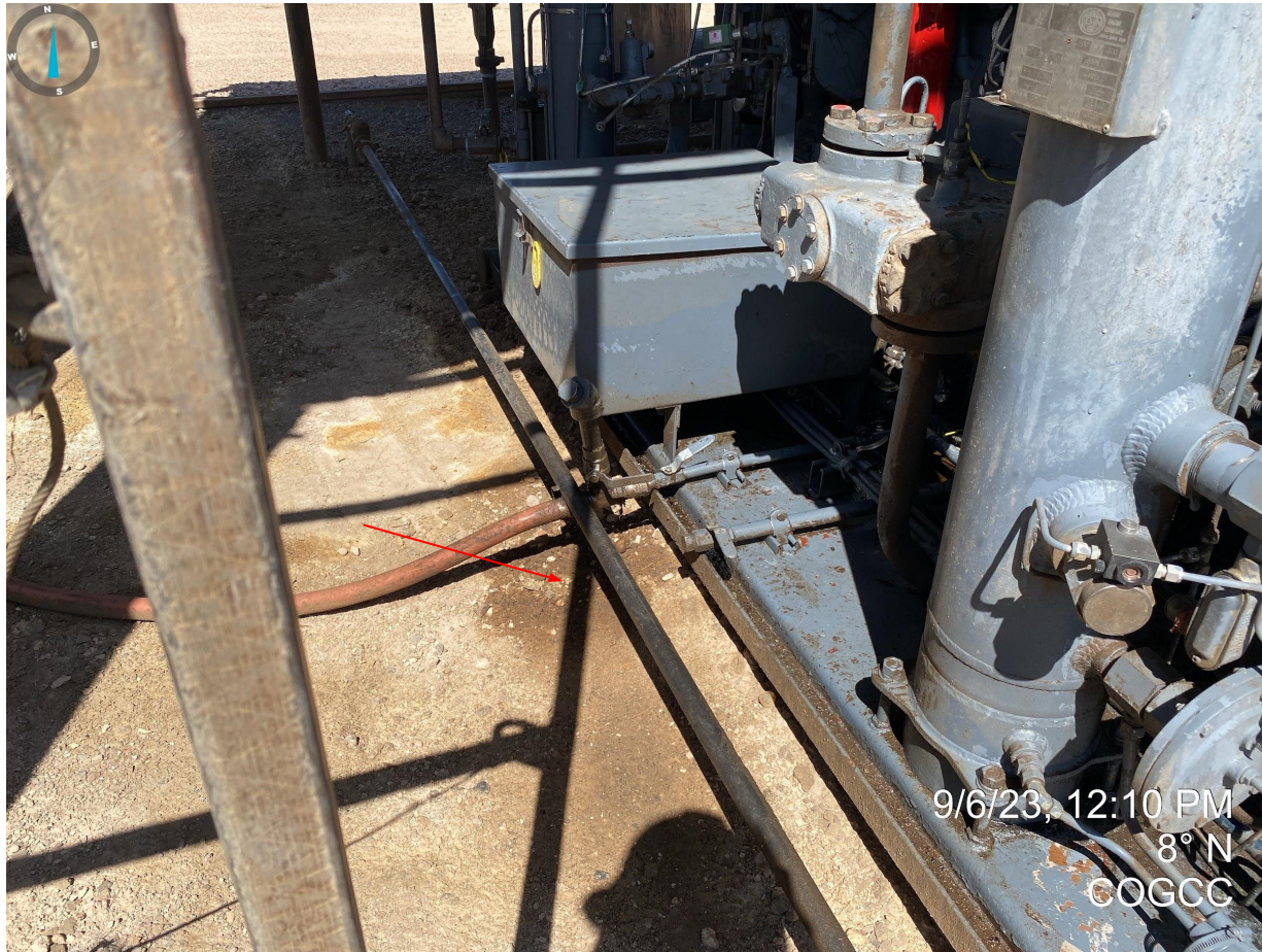
Photo 13. Stained soil observed at compressor.
