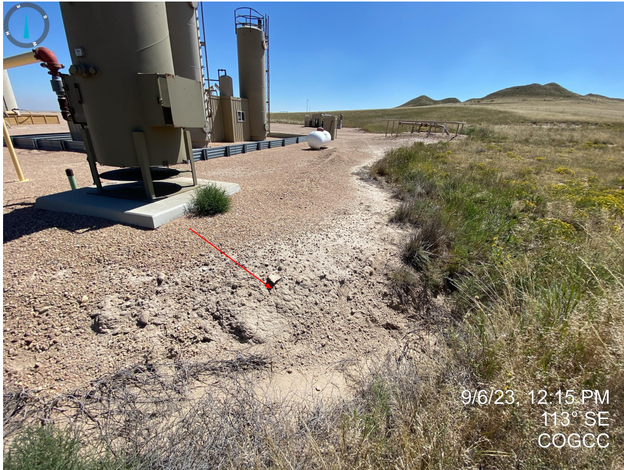
Photo 23. Production areas do not appear to be adequately stabilized with evidence of unconsolidated material. Taken from the southwest corner of the location.
