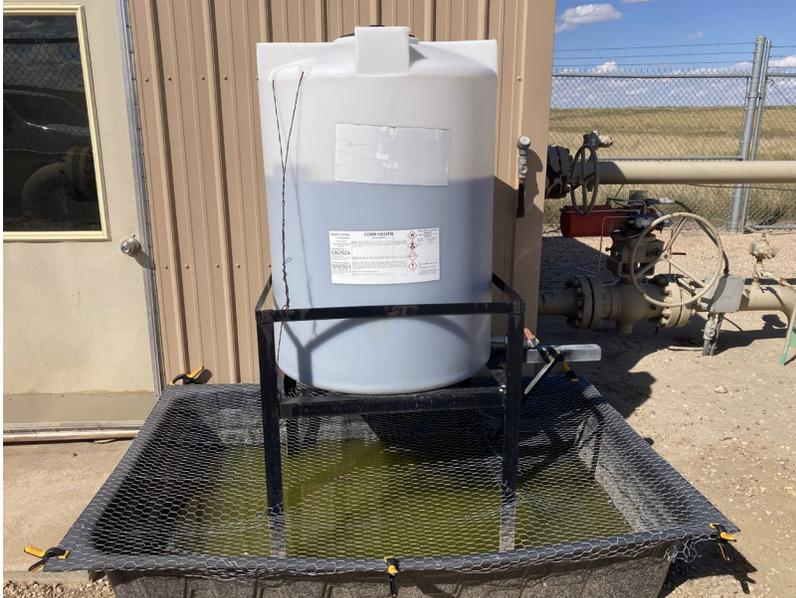
4) NFPA Placards on day tank and equipment are either missing, not legible, or peeling/faded/cracked. Refer to attached inspection photos for additional.
