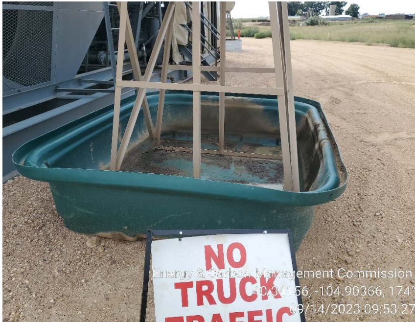
Bulk lube oil storage wildlife protection
