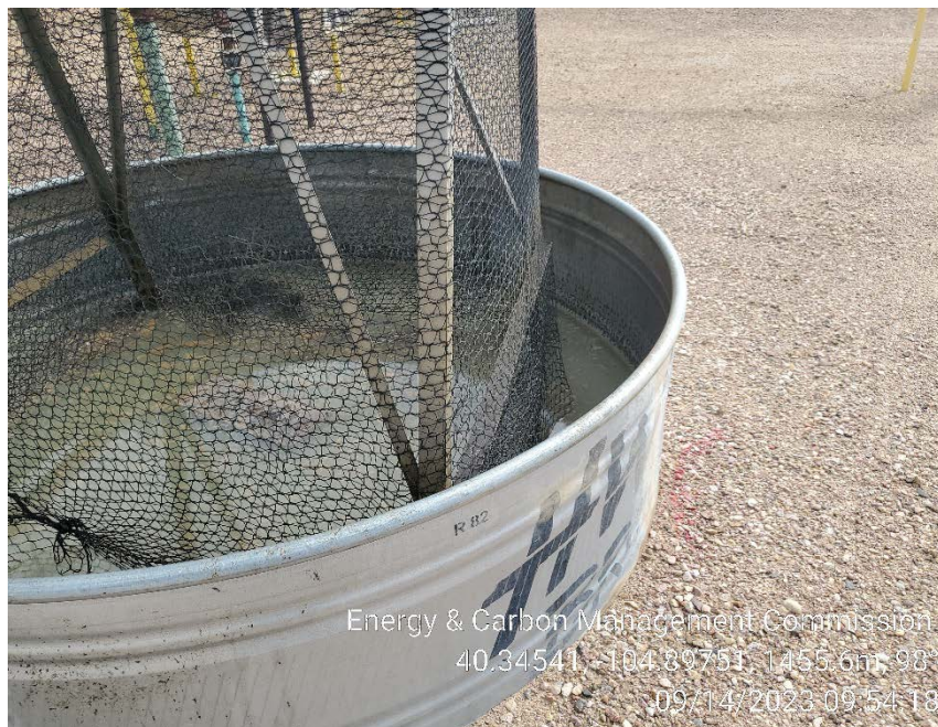
Bulk lube oil storage wildlife protection
