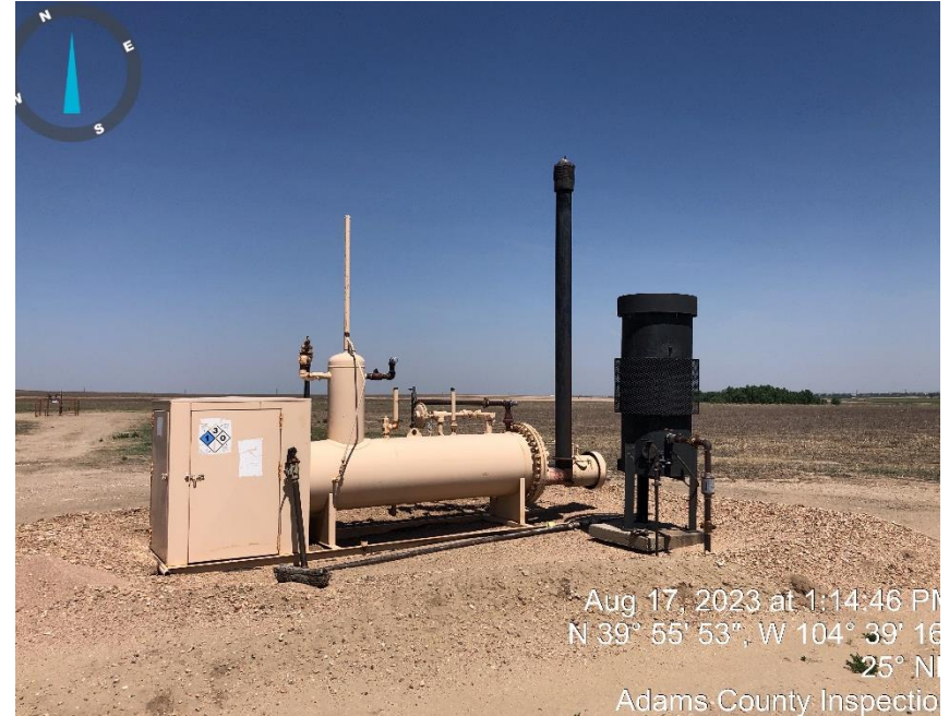
Photo #2 Separator and ECD.
