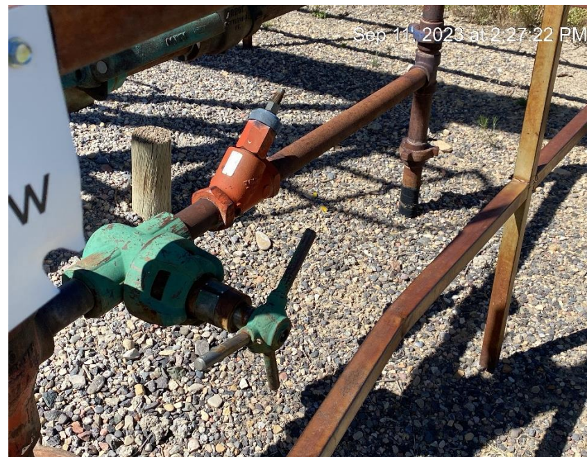
Casing venting directly to production tank
