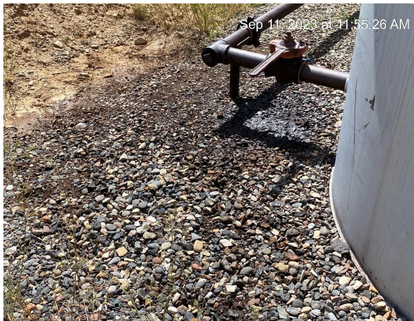
Leaking equipment. Staining.
