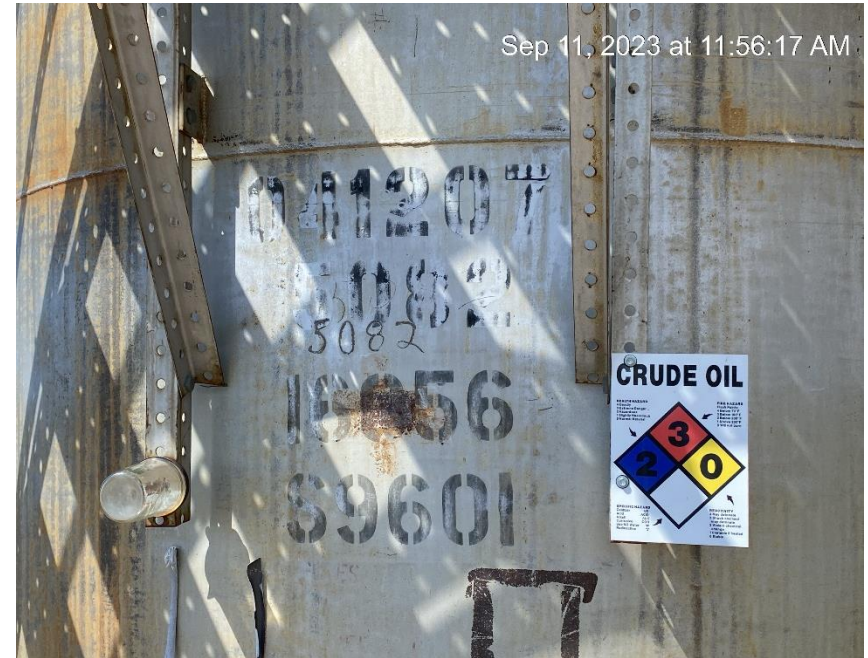
2 of 3 tanks missing Name of Operator and Operator's emergency contact number.
