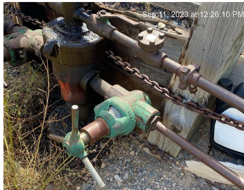
Casing venting to flowline
