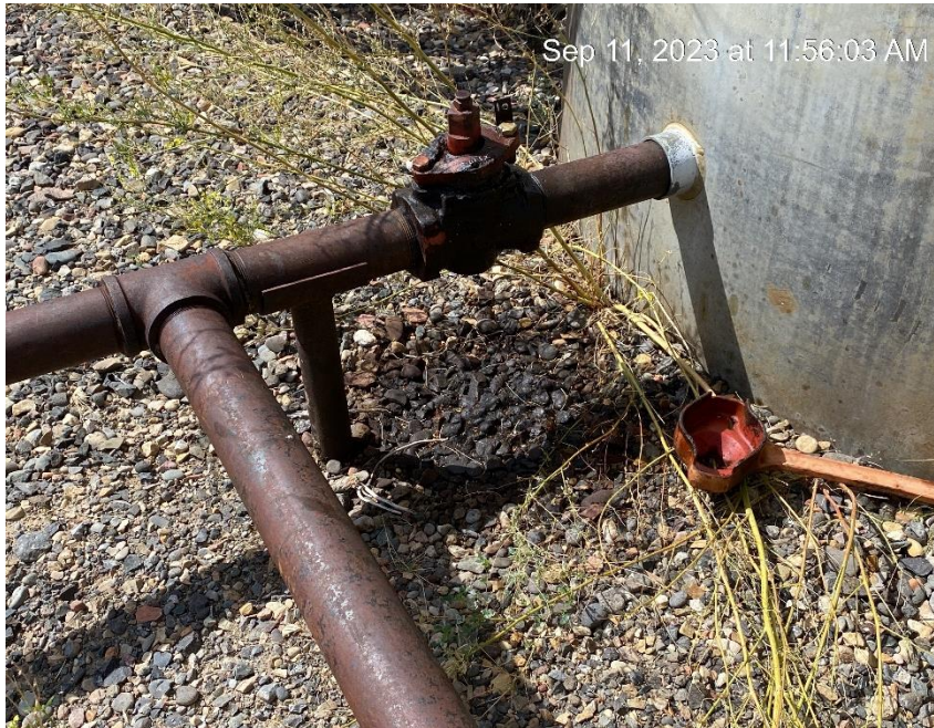
Leaking equipment. Staining. Debris
