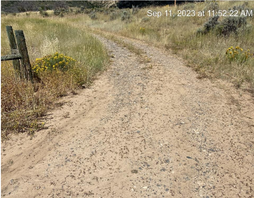
Access road at location. Insufficient Stormwater BMPs
