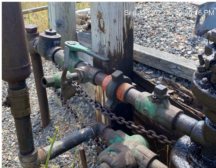
Flowline open to tank battery
