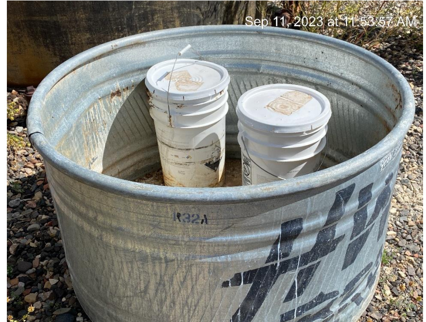
Open top tank lacking wildlife protection. Storage of chemicals
