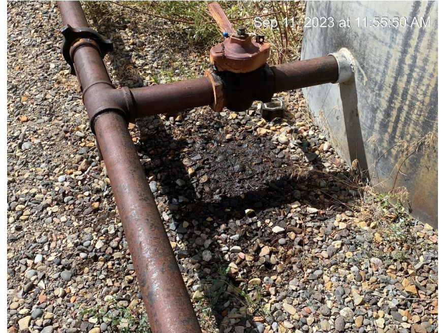
Leaking equipment, Staining.
