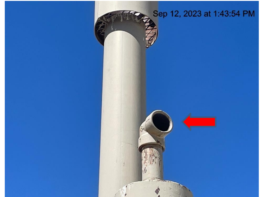
Photo # 8984 Open ended pipe/wildlife hazard
