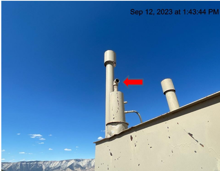
Photo # 8983 Open ended pipe/wildlife hazard
