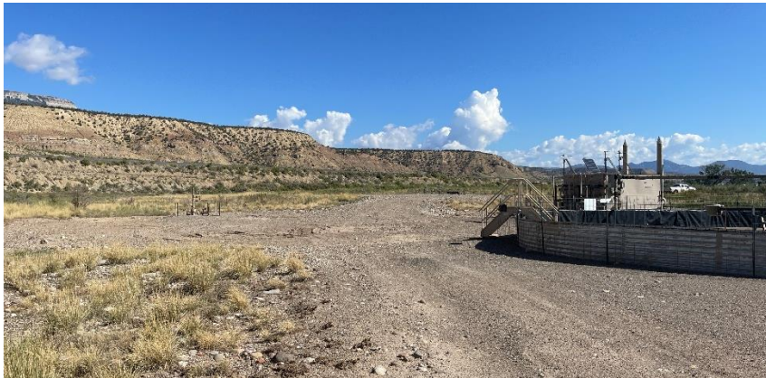
South West corner of location.
