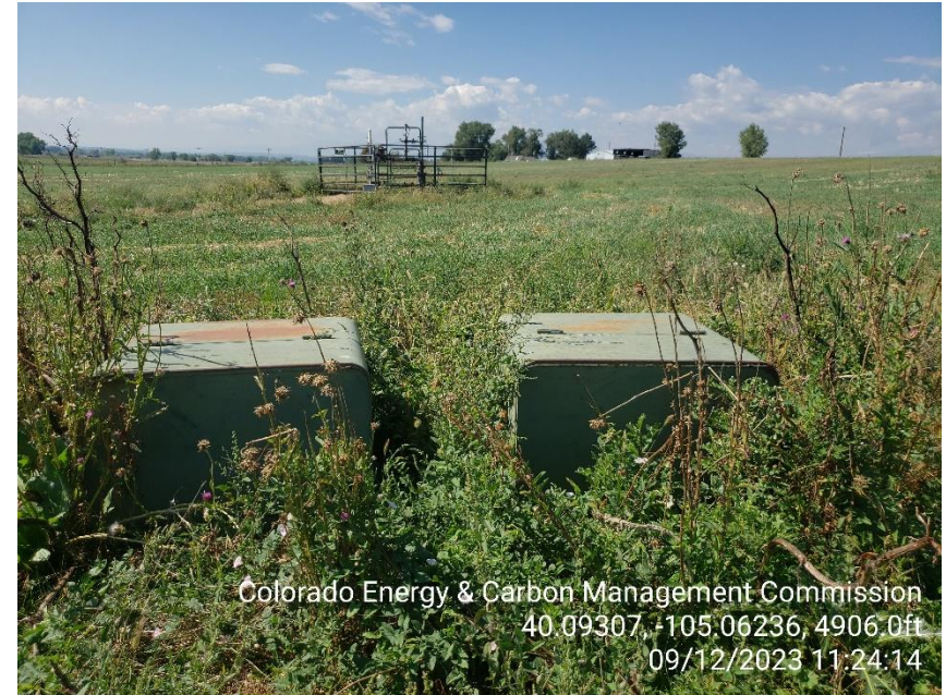
Photo 6 Undesirable vegetation growing tall around unused transformers.
