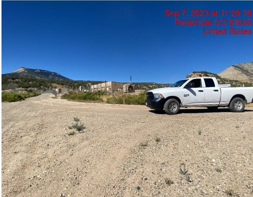
Insufficient Vehicle Tracking BMPs at Location Entrance/Exit – Photo #06330
