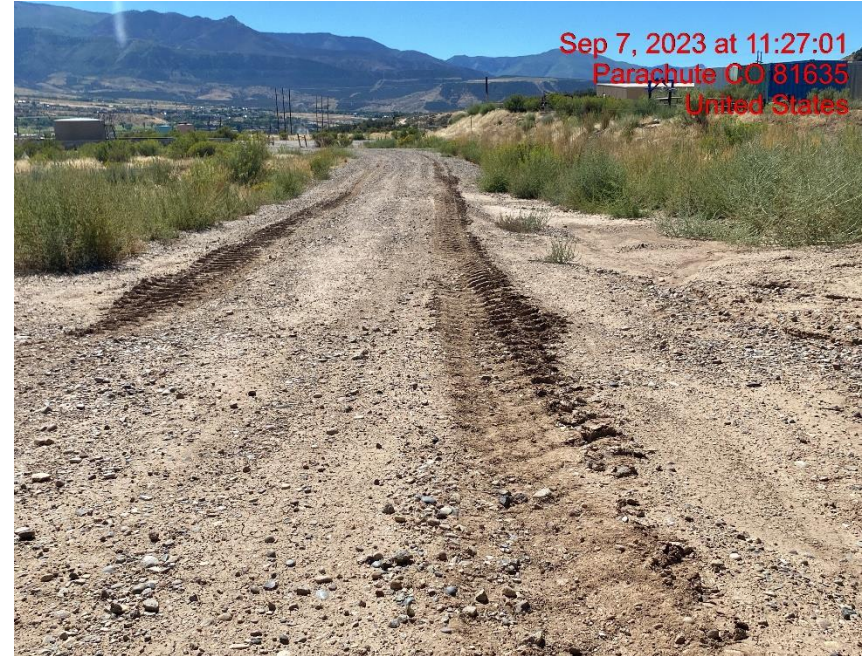
Access Road Lacks Stabilization – Photo #06329
