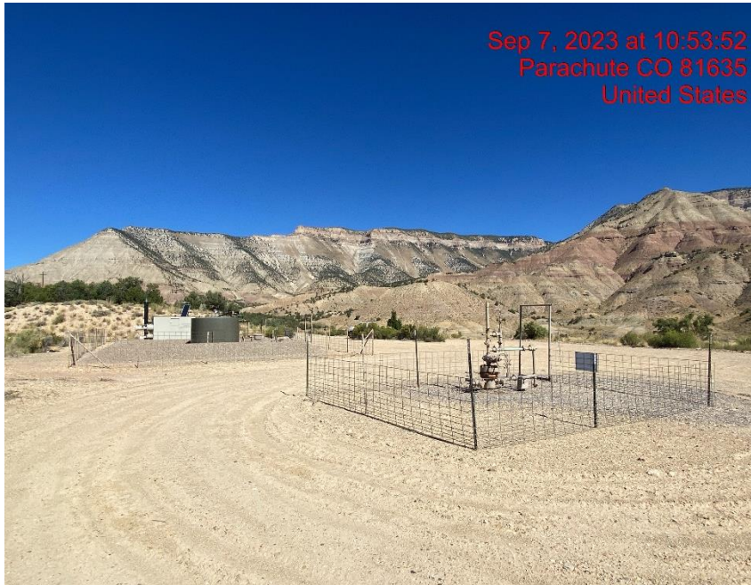
SW Corner of Location – Photo #06301
