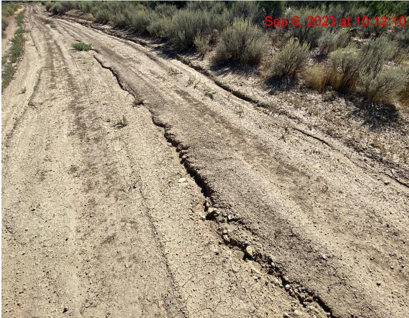
Access Road Lacks Stabilization – Photo #06269
