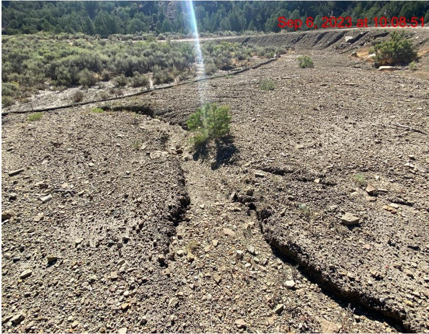
Rill Erosion Transporting Sediment Off-Location – Photo #06258
