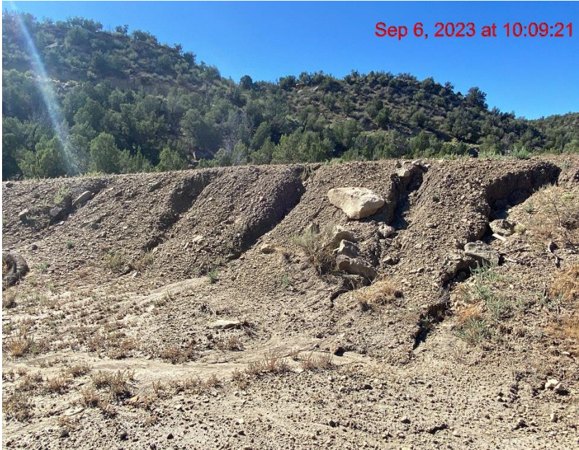
Gulley Erosion Transporting Sediment Off-Location – Photo #06261
