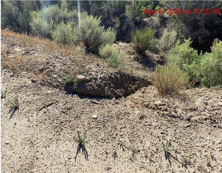
Rill Erosion Transporting Sediment from Access Road to Drainage Ditch – Photo #06265
