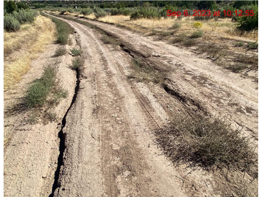
Access Road Lacks Stabilization – Photo #06270
