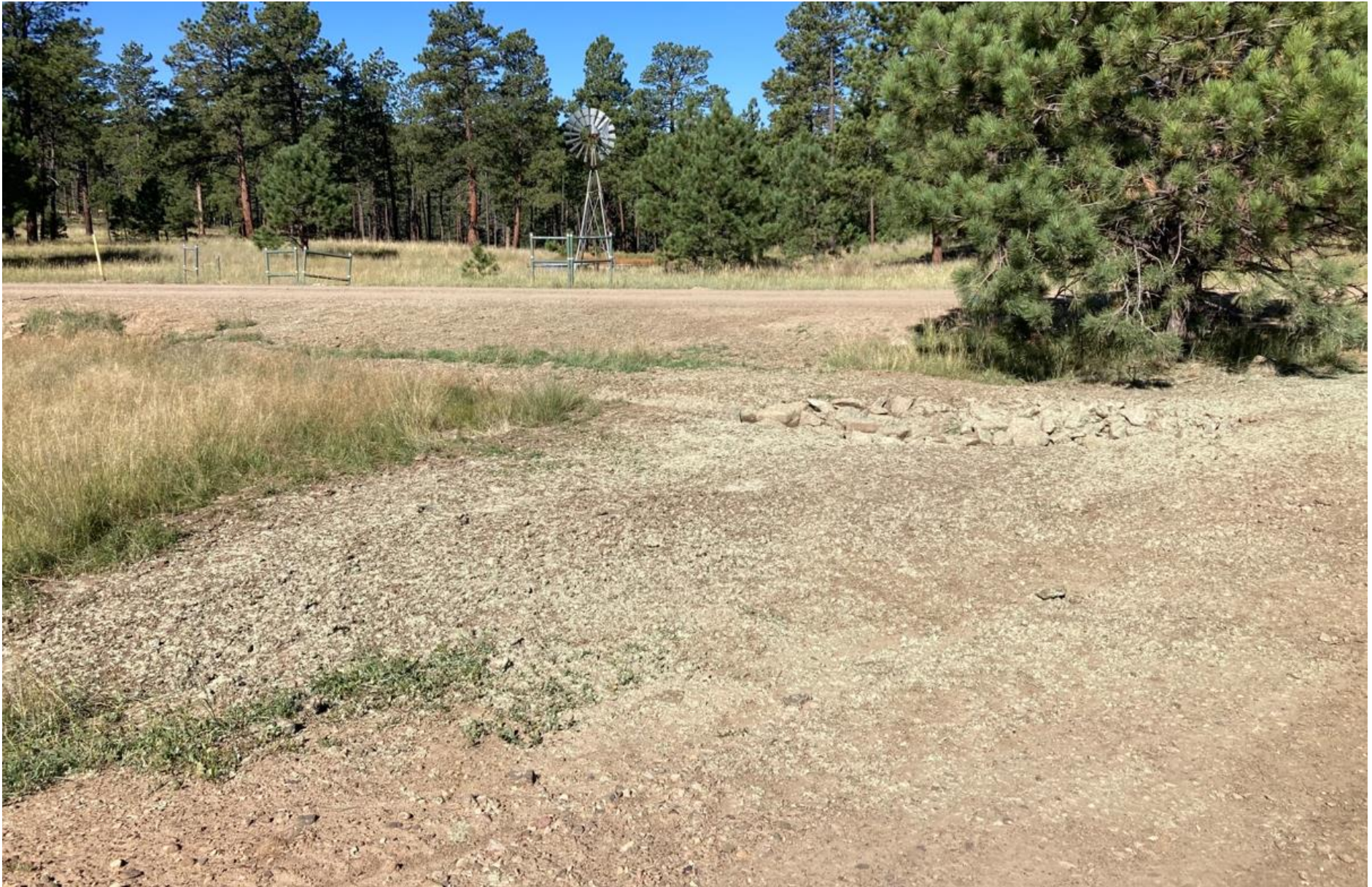
PHOTO 7: ROCKED OUTLET AND DIVERSION DITCH. THIS AREA IS ALSO RELATED TO INSPECTION DOC #713600179 AND FIRR DOC #403521679. THE DISTURBED AREA HAS BEEN THOROUGHLY HYDRO-MULCHED AND SEEDED POST REMOVAL OF ROCK STOCK PILE.
