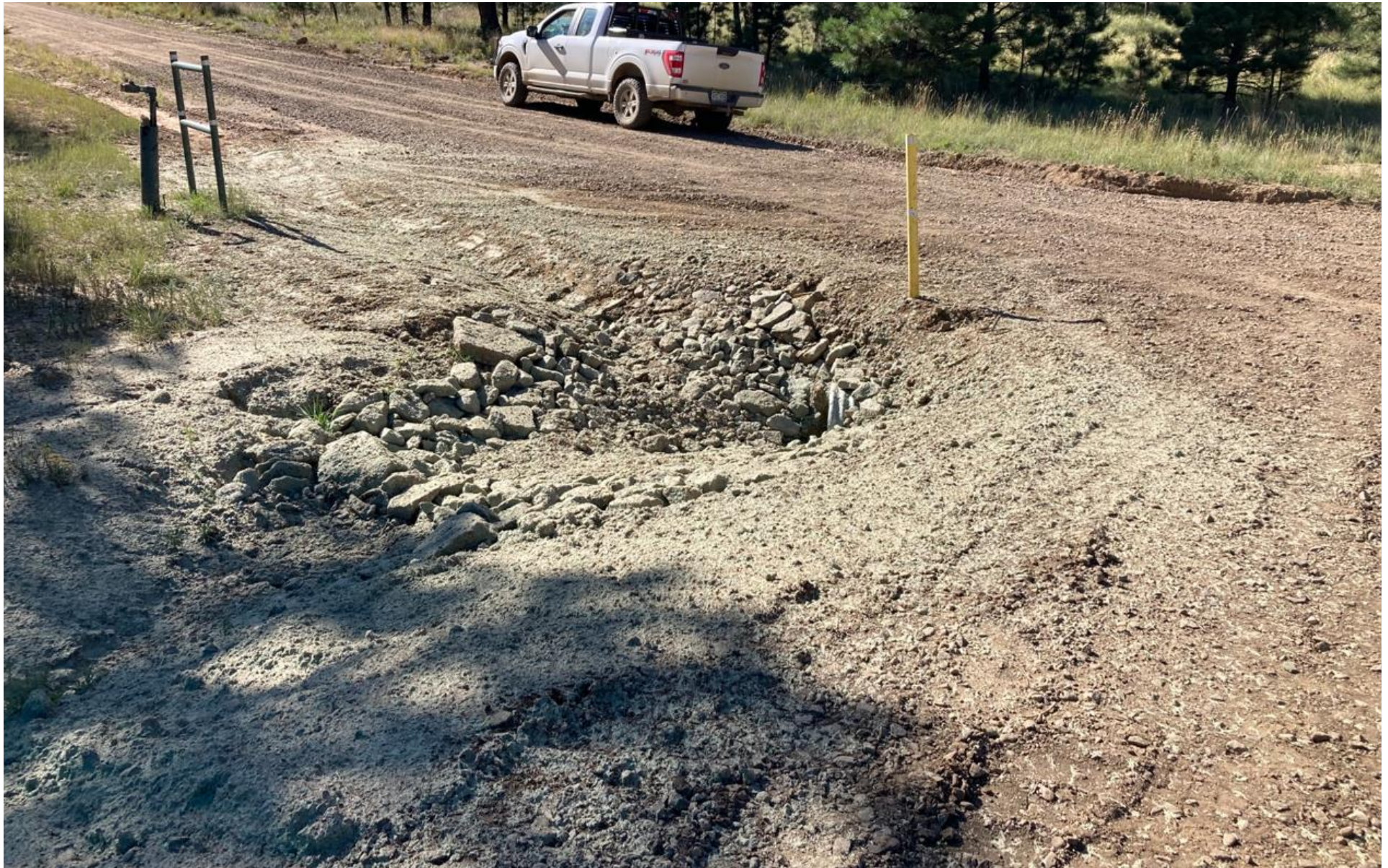
PHOTO 2: A CULVERT HAS BEEN INSTALLED AT THE INTERSECTION IDENTIFIED IN DOC #690203935 TO PROPERLY DIVERT STORMWATER. BOTH THE INLET AND OUTLET HAVE BEEN DEFINED AND ROCKED. ALL DISTURBED AREAS HAVE BEEN SEEDED TO PROMOTE VEGETATIVE STABILIZATION.
