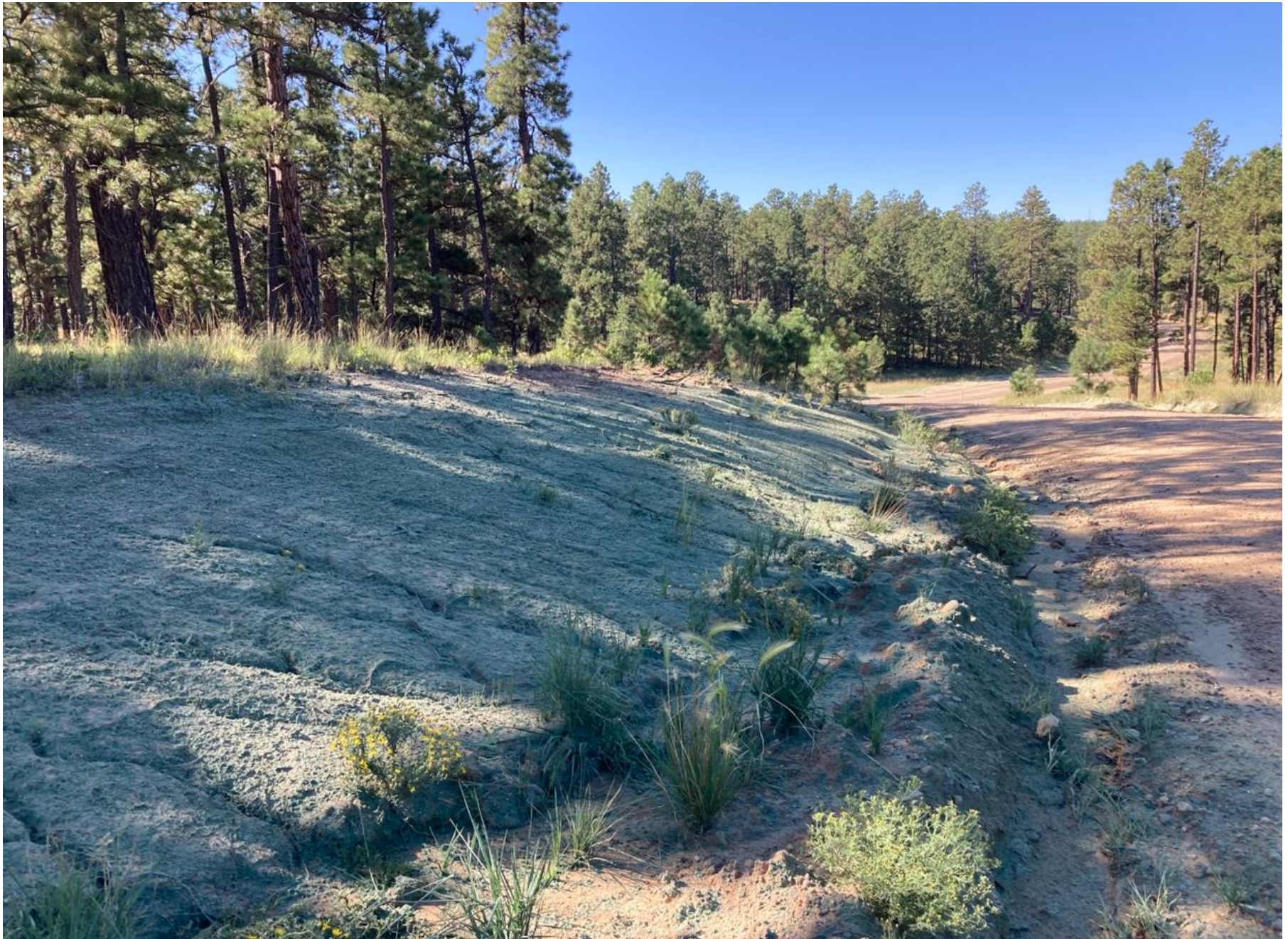
PHOTO 1: THE CUT SLOPE IDENTIFIED IN DOCUMENT #690203935 HAS BEEN SEEDED TO ESTABLISH STABILIZATION.
