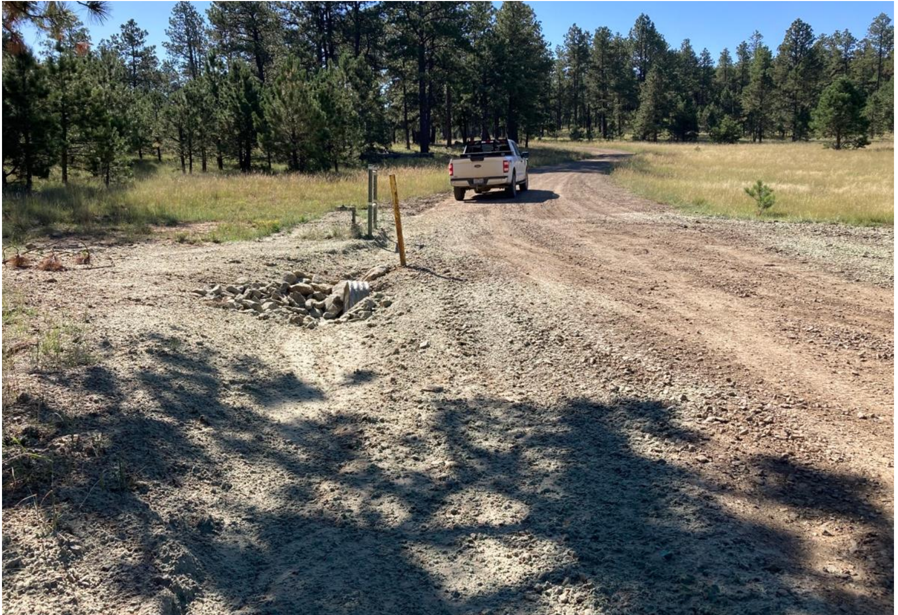
PHOTO 5: ALL CULVERTS IN THE AREA ASSOCIATED WITH THE INITIAL CORRECTIVE ACTION HAVE BEEN CLEANED OF SEDIMENT ACCUMULATION TO ALLOW PROPER FLOW THROUGH THE CULVERT. INLETS AND OUTLETS HAVE BEEN REDEFINED/ROCKED. ALL DISTURBED AREAS HAVE BEEN HYDRO-MULCHED AND SEEDED TO PROMOTE VEGETATIVE STABILIZATION. THE AREA WILL BE FURTHER MONITORED FOR GROWTH, NOXIOUS WEEDS, SEDIMENT MOVAL AND STORMWATER IMPACT.
