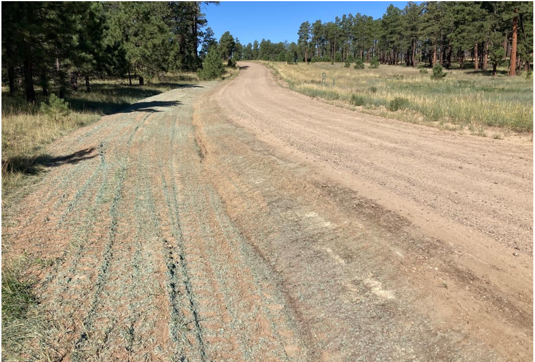
PHOTO 4: THE BAR DITCH THROUGHOUT THE AREA HAS BEEN RECONFIGURED TO ELIMINATE EROSION AND THE SOIL WAS COMPACTED AND TRACKED FOR STABILIZATION. ALL DISTURBED AREAS HAVE BEEN HYDRO-MULCHED & SEEDDED.
