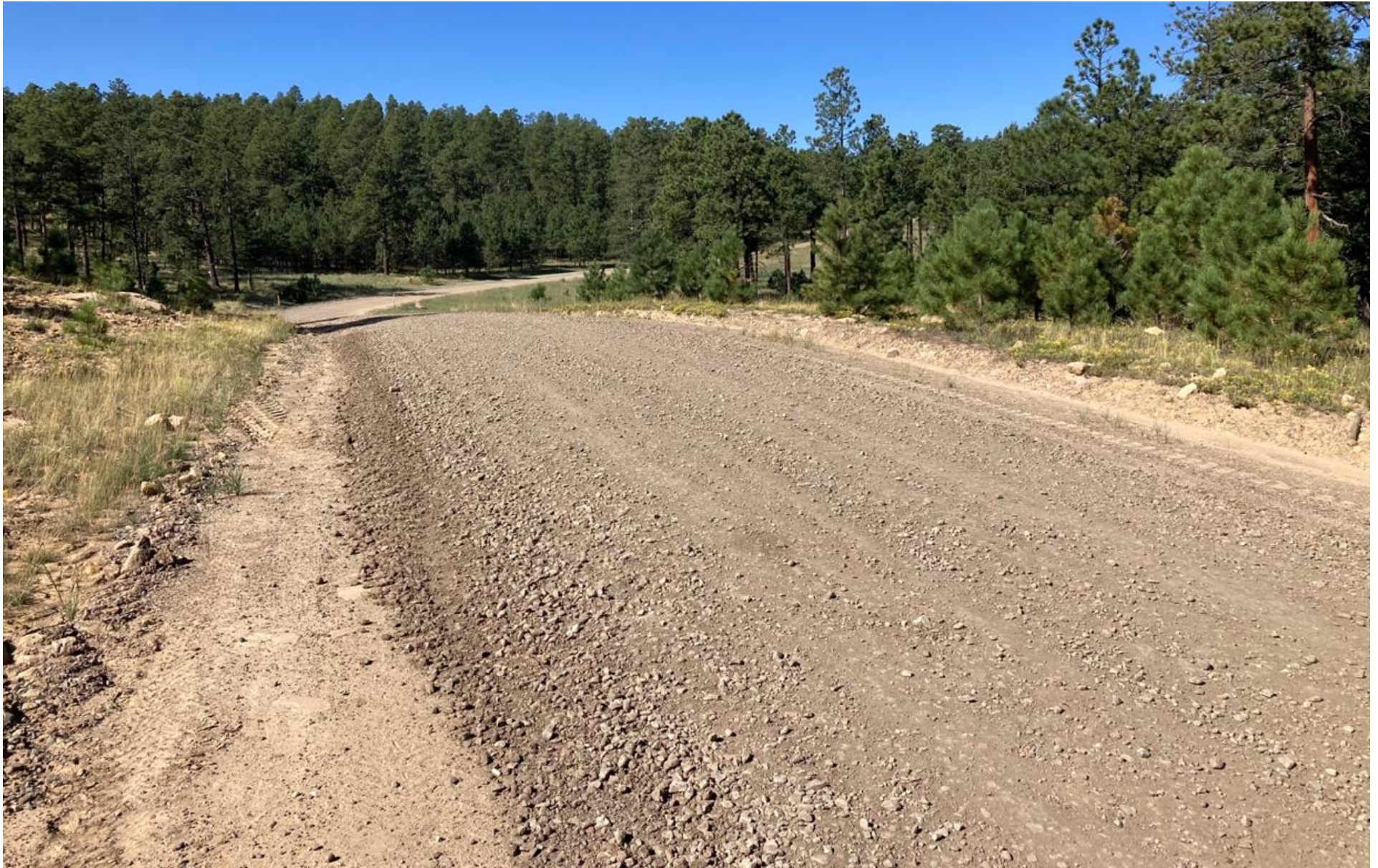
PHOTO 13: THE ROAD SURFACE WAS CROWNED THROUGHOUT THE AREA TO CREATE SHEET FLOW AND ELIMINATE THE TIRE RUTS. ADDITIONAL GRAVEL MATERIAL WAS INSTALLED TO THE ROADWAY SURFACE TO PROVIDE ADDED STABILIZATION.
