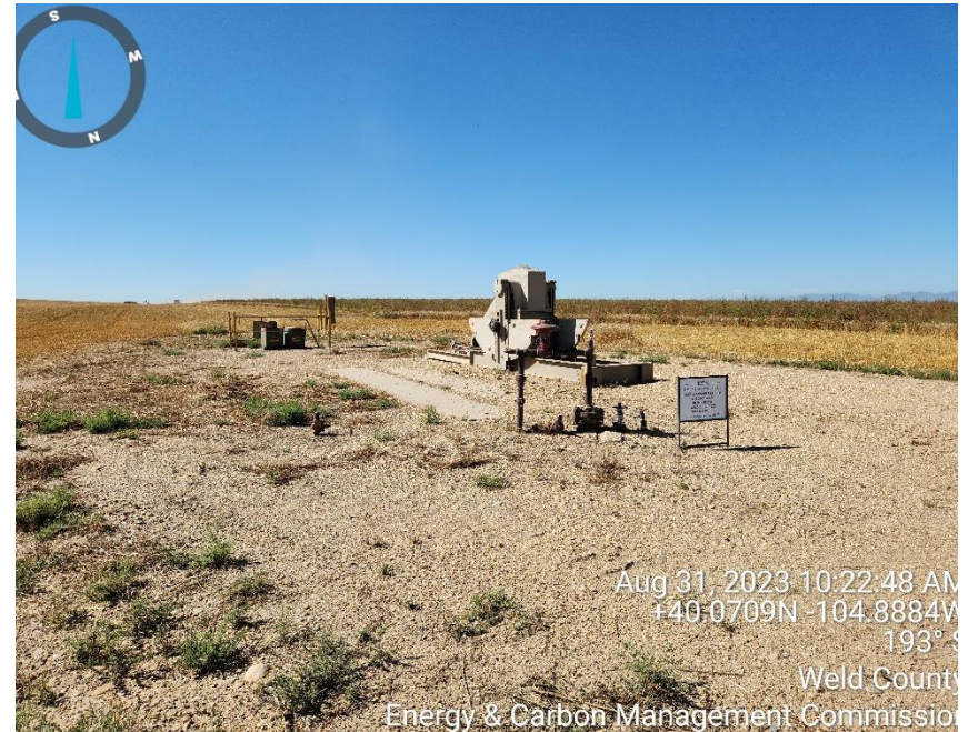
Photo 2 well head and unused equipment
