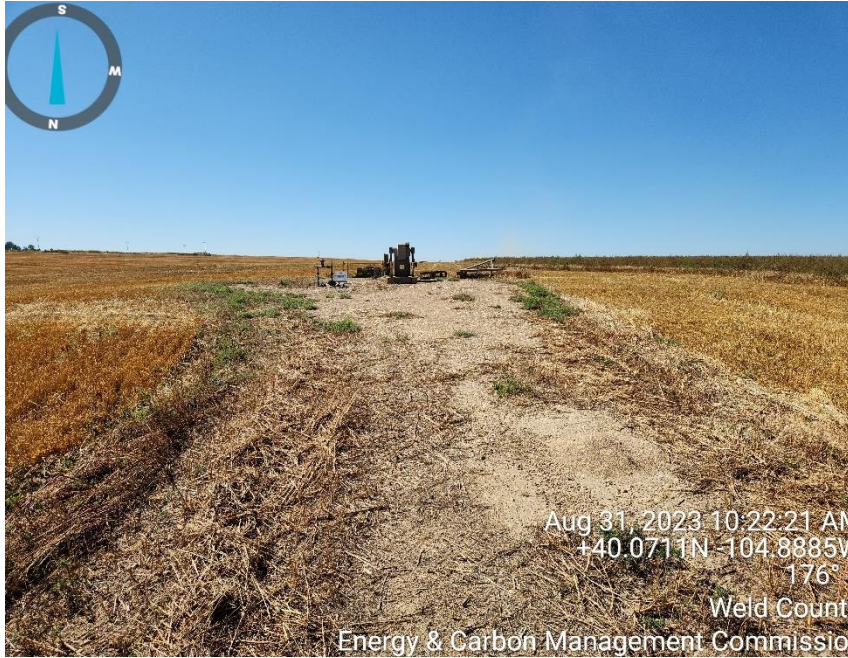
Photo 1 access road, well head and unused equipment
