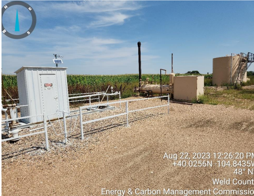
Photo 5 meter run and separator
