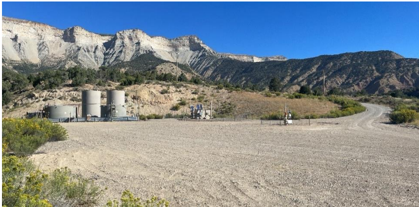
South West corner of location.
