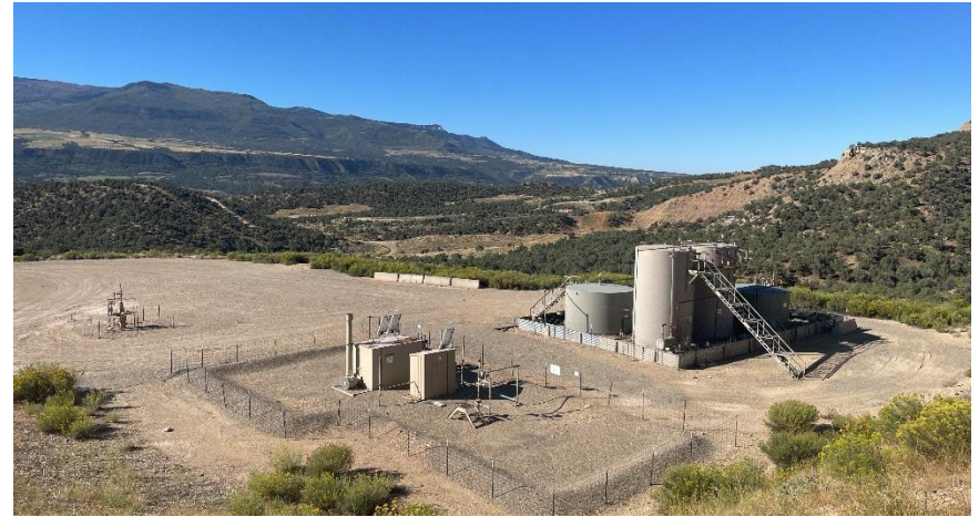
North East corner of location.
