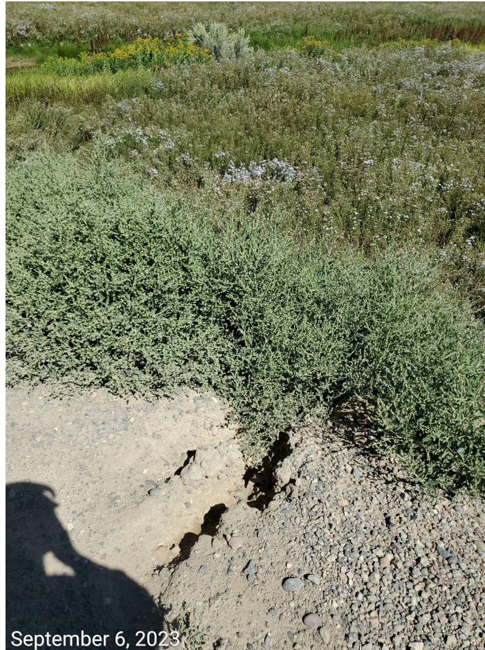
Photo 9: Photo example showing erosion degradation along access road
