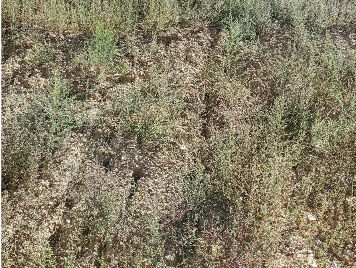
Photo 7: Erosion degradation on cut slopes.
