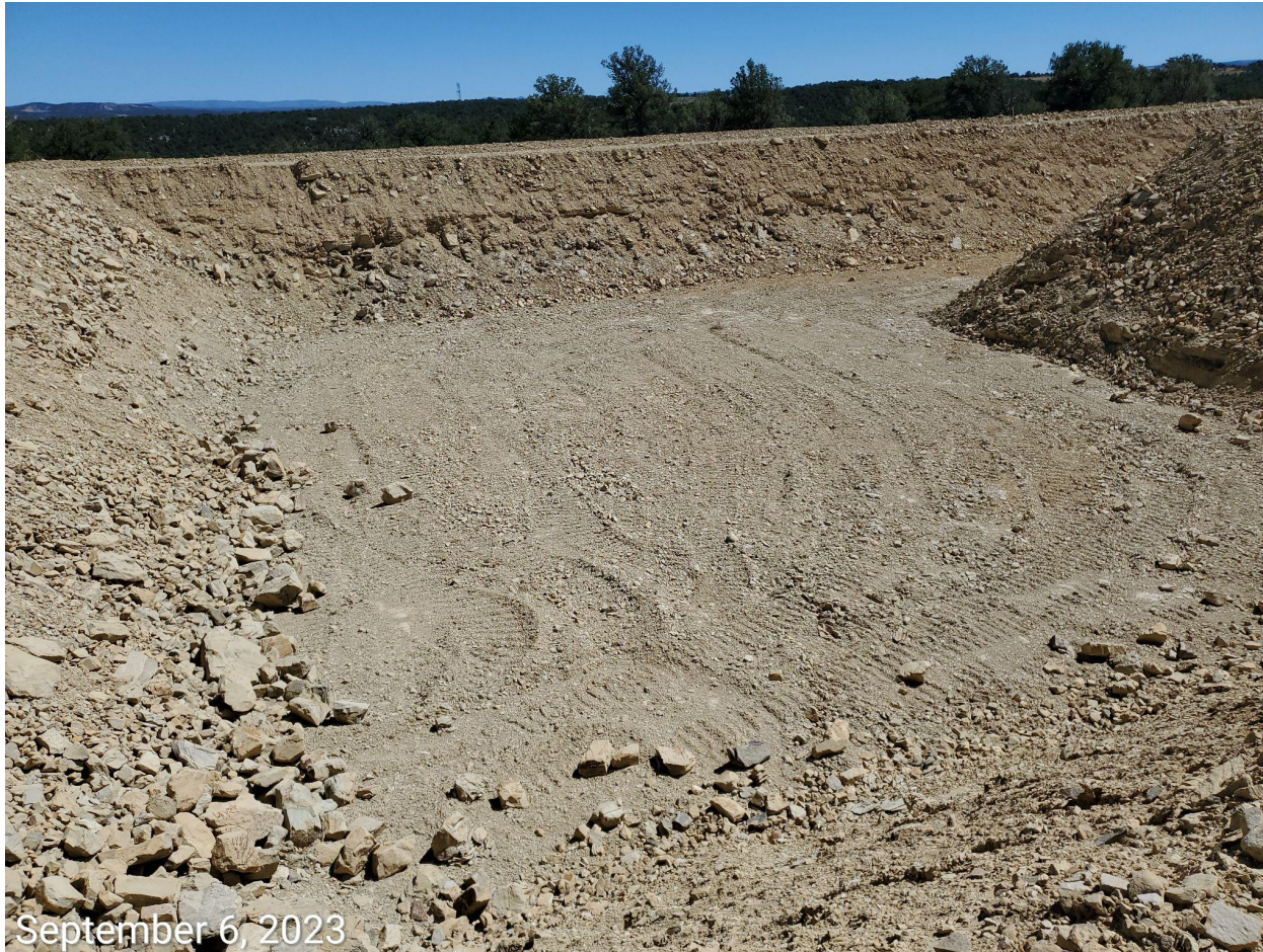
Photo 4: Cuttings trench has been constructed.
