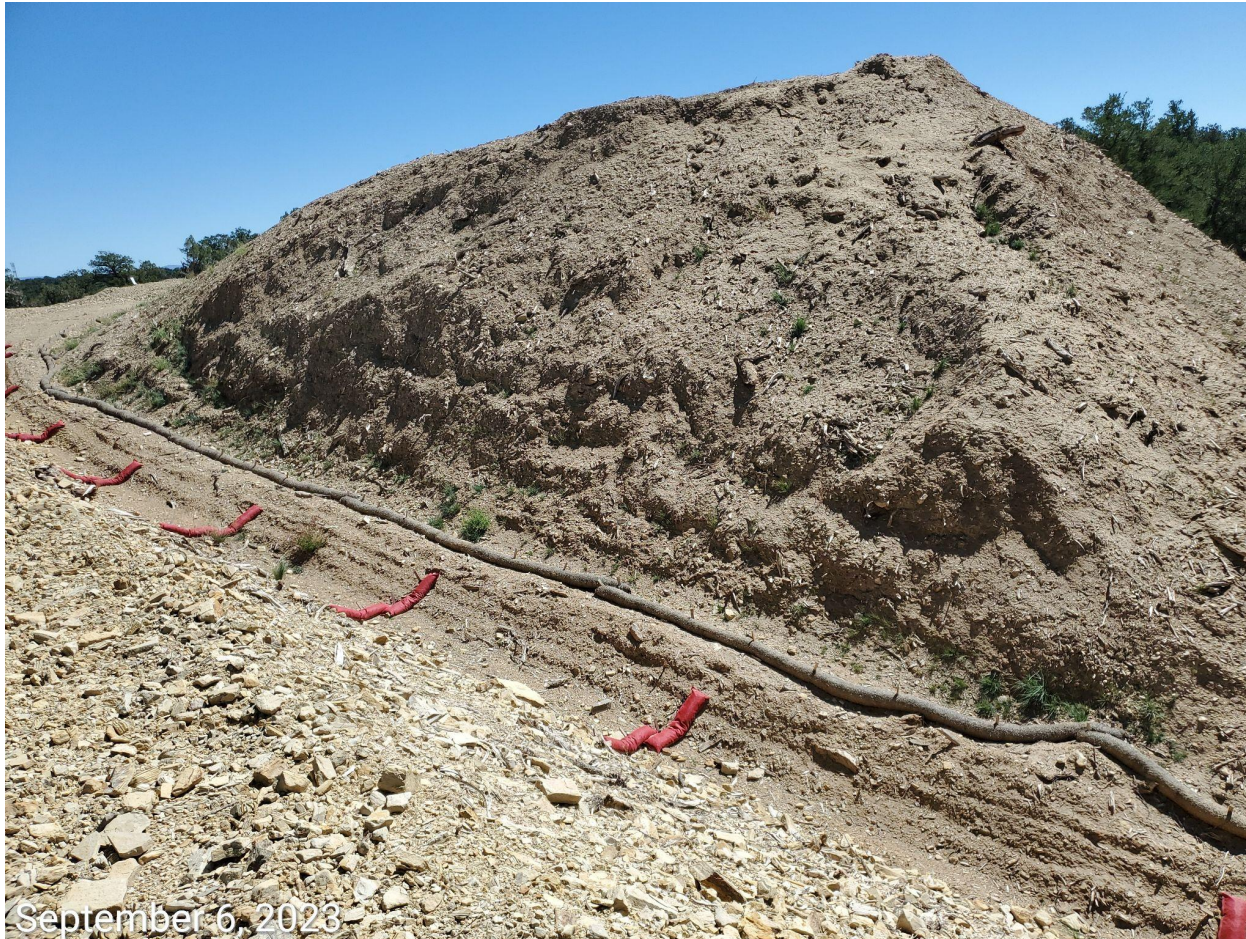
Photo 3: Hydromulch along steep sections of the topsoil stockpile show signs of disrepair.
