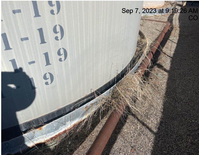
Photo # 8447 Weeds/undesirable plant species in secondary containment
