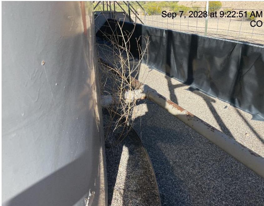
Photo # 8457 Weeds/undesirable plant species in secondary containment
