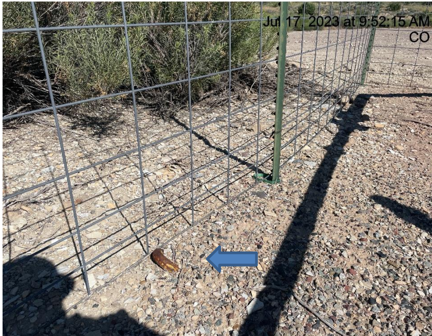
Photo # 3158 From inspection 708901066 conducted on 07/17/2023 Unmarked deadman/anchor
