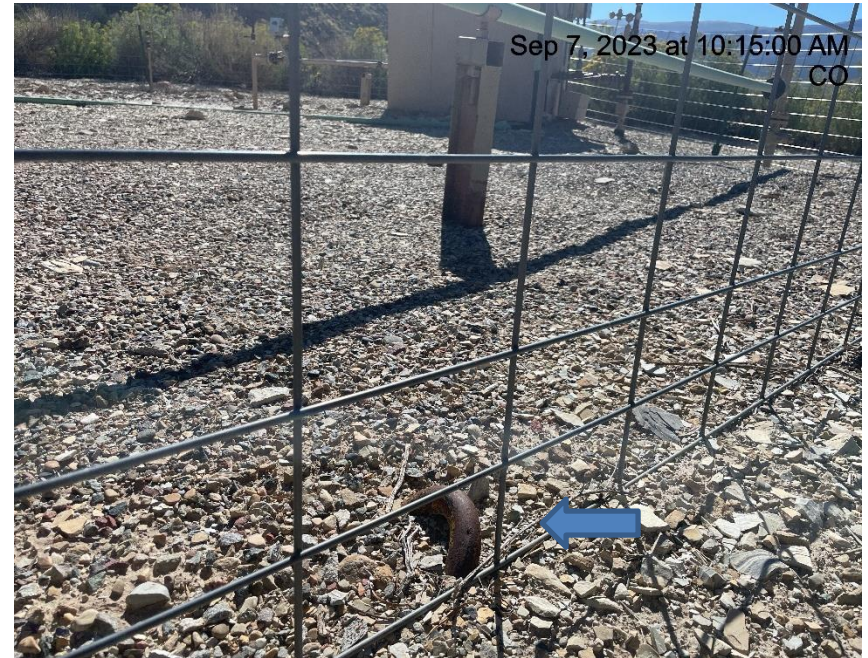
Photo # 8527 Same unmarked deadman/anchor from a different angle
