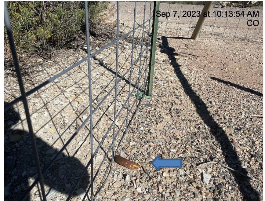
Photo # 8522 Unmarked deadman/anchor
