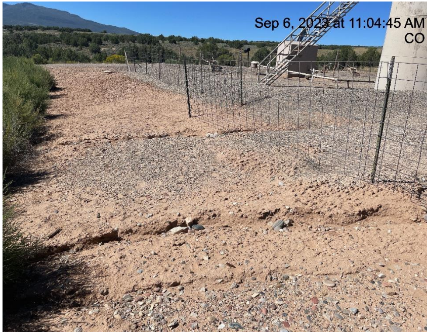
Photo # 8341 Erosion & transport of sediment off location & into a vegetated area/BMP's need maintenance
