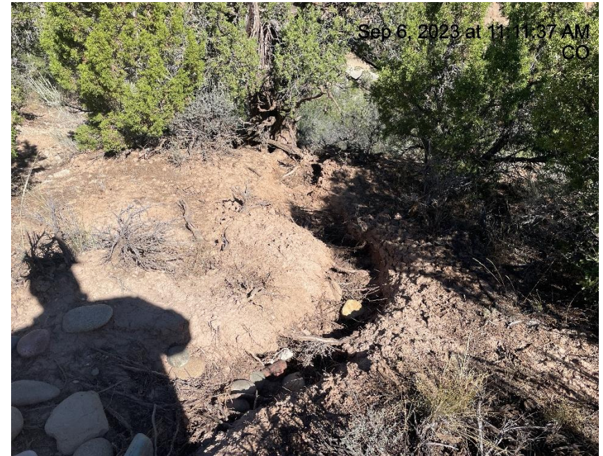
Photo # 8368 Rip Rap/BMP's need maintenance/erosion & transport of sediment/insufficient runoff controls/BMP's (NW corner of location after sediment trap)
