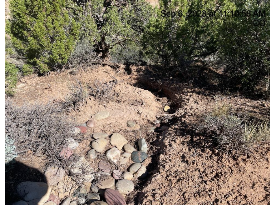
Photo # 8364 Rip Rap/BMP's need maintenance/erosion & transport of sediment/insufficient runoff controls/BMP's (NW corner of location after sediment trap)
