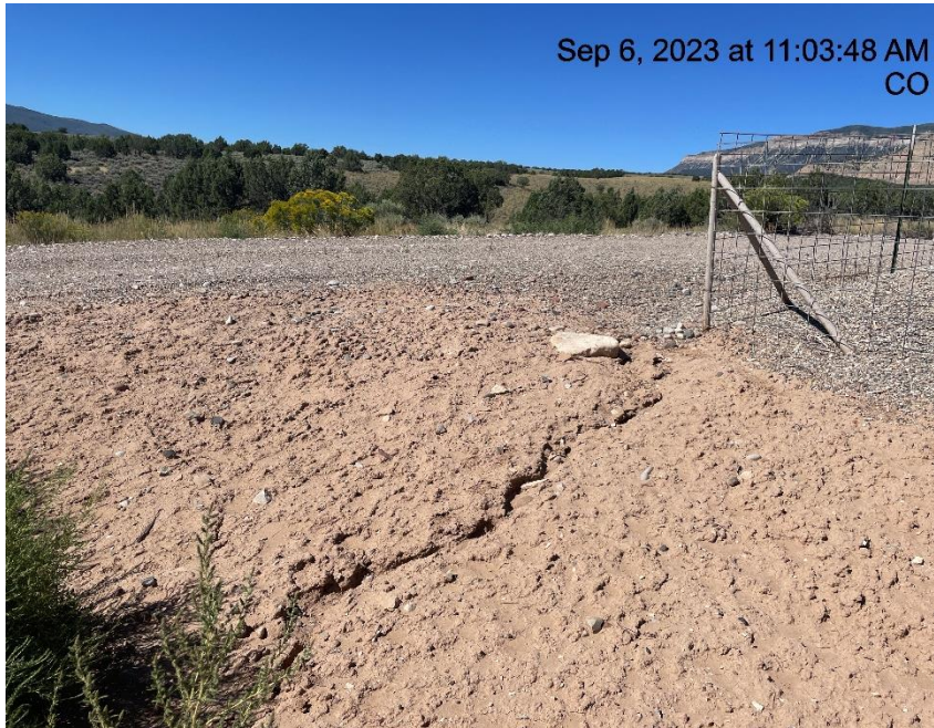
Photo # 8336 Erosion & transport of sediment off location & into a vegetated area
