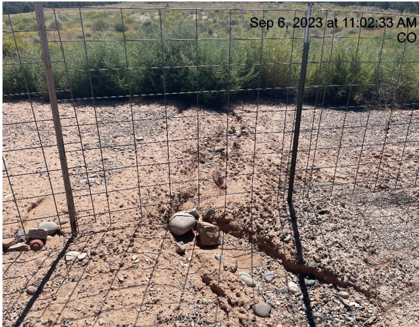
Photo # 8331 Erosion & transport of sediment off location & into a vegetated area/BMP's need maintenance
