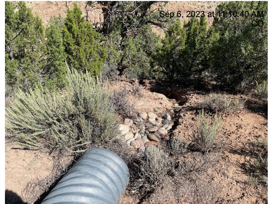
Photo # 8362 Rip Rap/BMP's need maintenance/erosion & transport of sediment/insufficient runoff controls/BMP's (NW corner of location after sediment trap)
