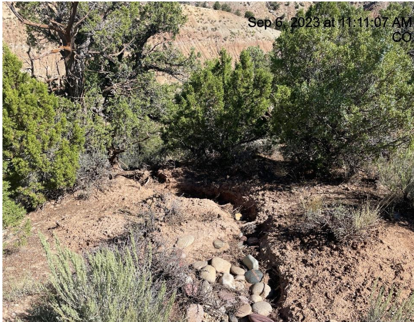
Photo # 8365 Rip Rap/BMP's need maintenance/erosion & transport of sediment/insufficient runoff controls/BMP's (NW corner of location after sediment trap)
