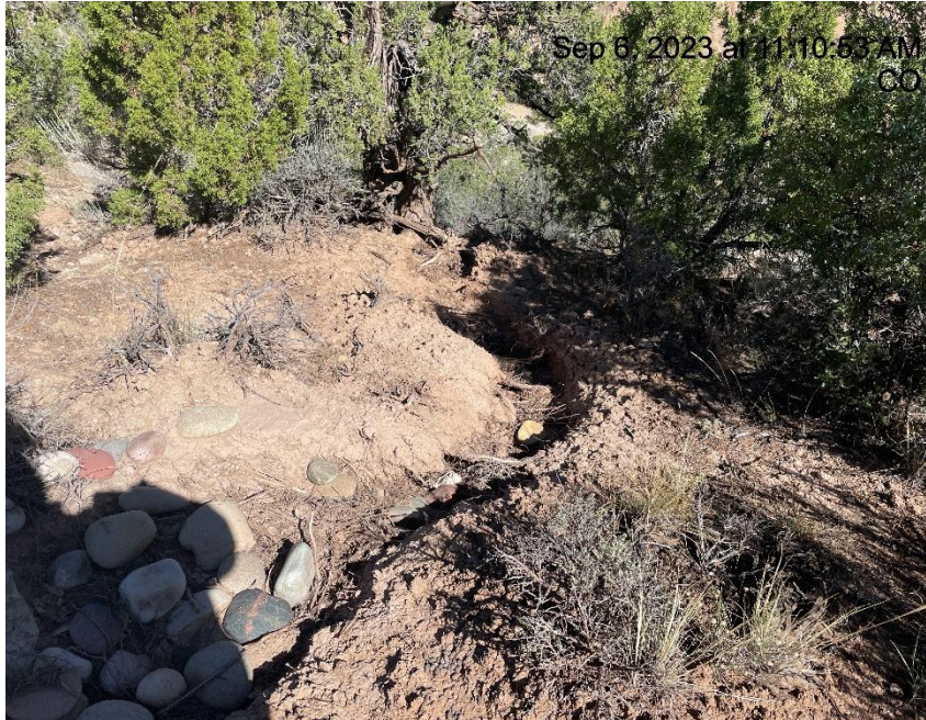
Photo # 8363 Rip Rap/BMP's need maintenance/erosion & transport of sediment/insufficient runoff controls/BMP's (NW corner of location after sediment trap)
