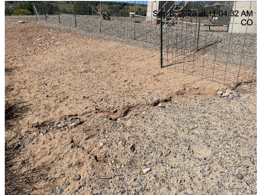
Photo # 8340 Erosion & transport of sediment off location & into a vegetated area/BMP's need maintenance
