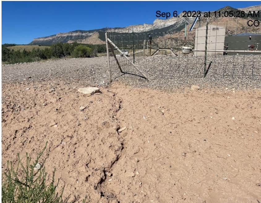
Photo # 8344 Erosion & transport of sediment off location & into a vegetated area
