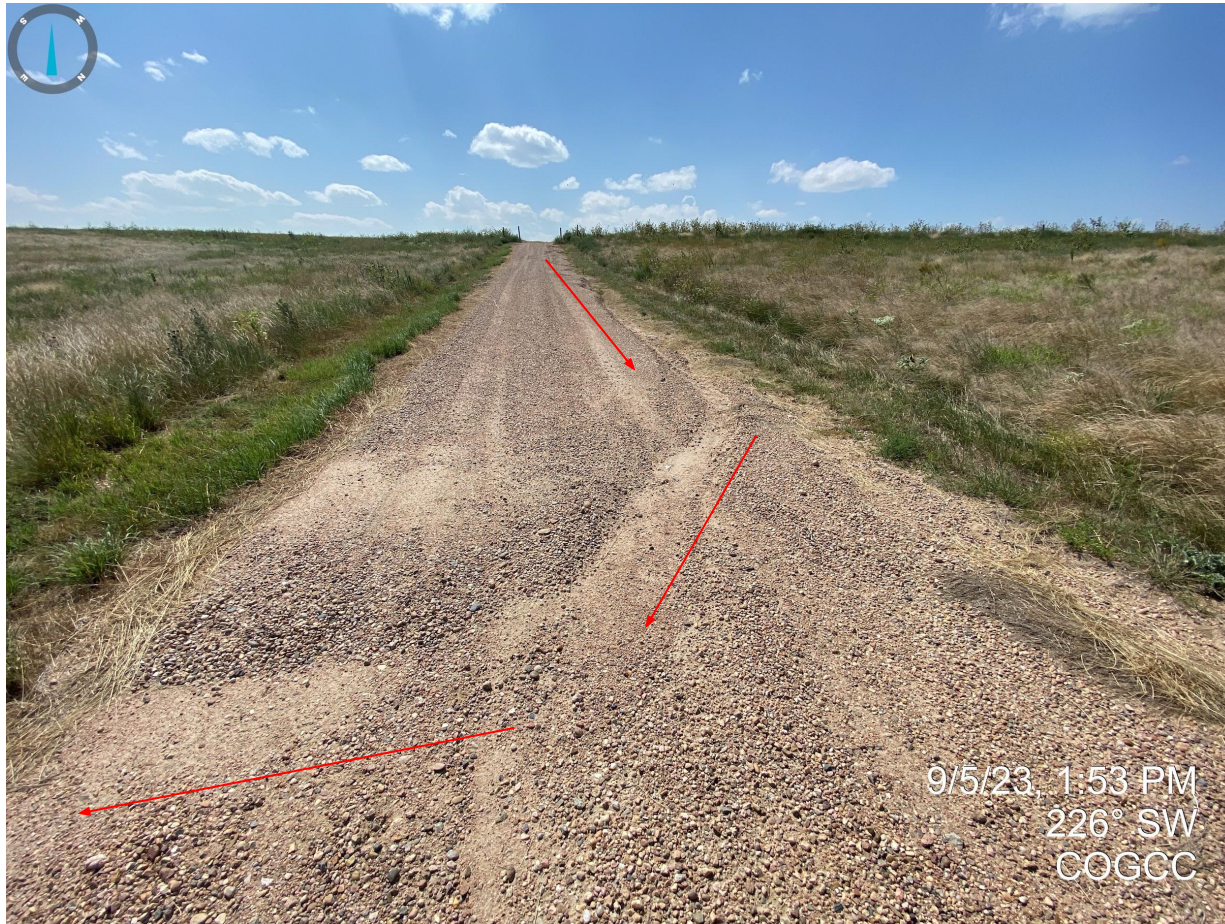
Photo 5. Rill erosion degradation occurring on the access roads. No apparent stormwater controls/BMPs were observed to prevent sediment from exiting off location.
