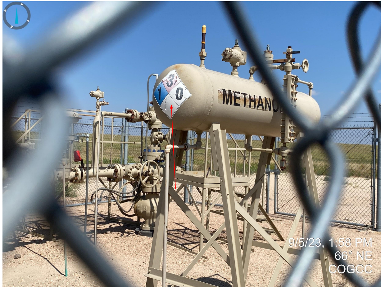
Photo 9. NFPA placard is faded/peeling/cracked and requires replacement.
