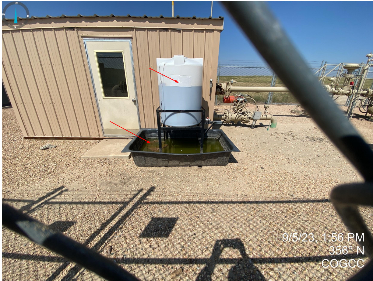
Photo 8. Day tank without legible labels and no wildlife protection/exclusion device installed around secondary containment.
