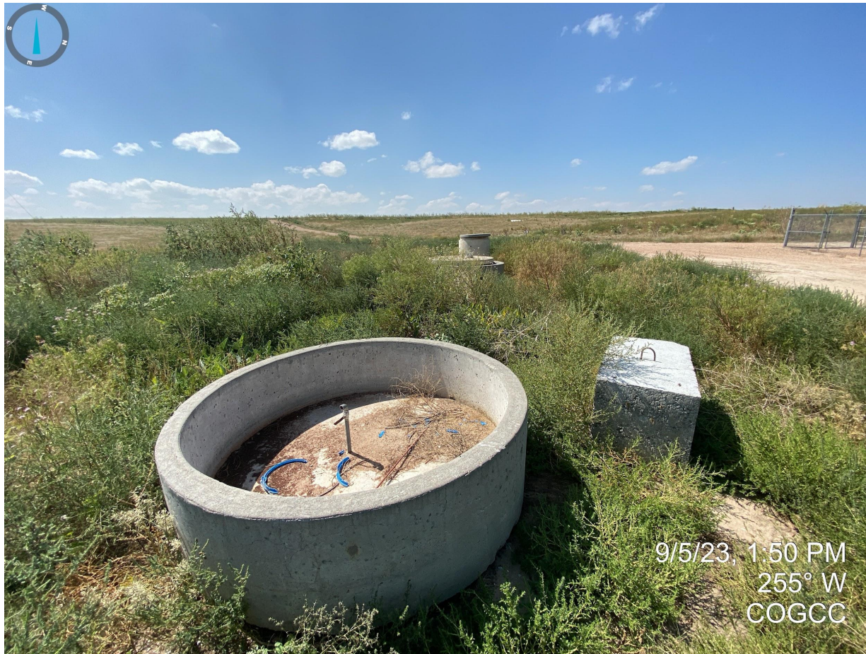
Photo 3. Concrete structures on location do not appear to be used and require removal per Rule 606.
