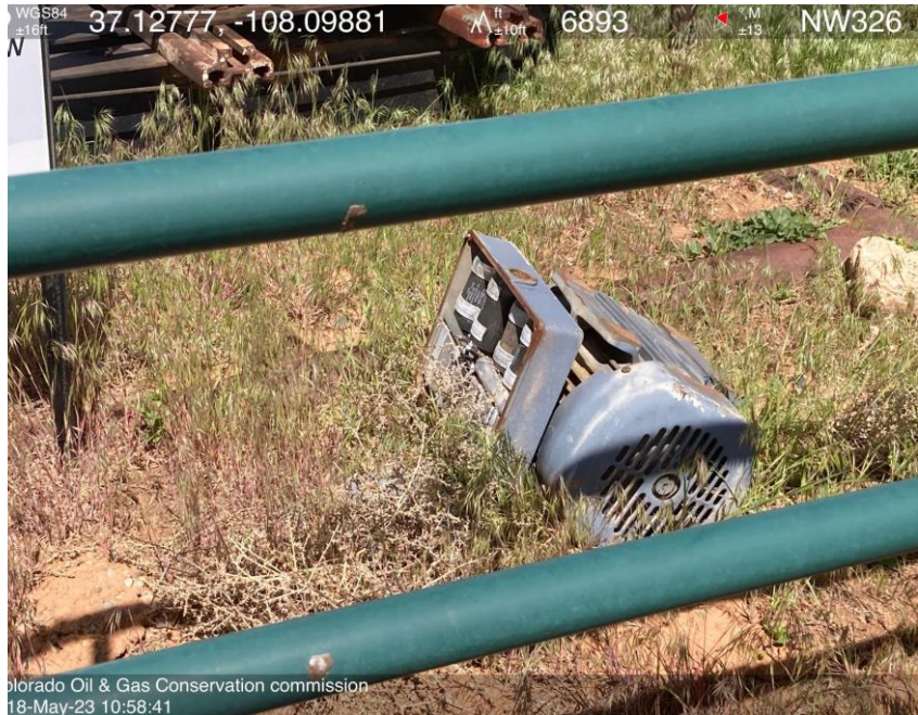
Photo #3. View of Corrective Action identified in FIR Doc.#695108244.
