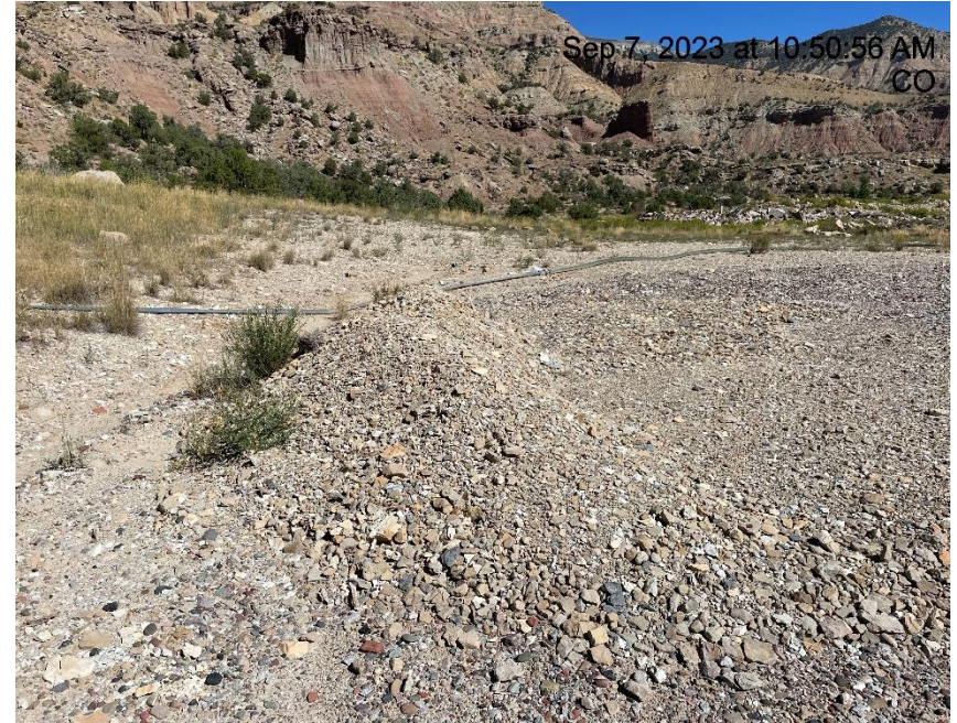
Photo # 8573 Stockpiled soils/insufficient BMP's
