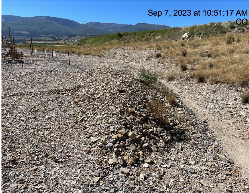
Photo # 8574 Stockpiled soils/insufficient BMP's
