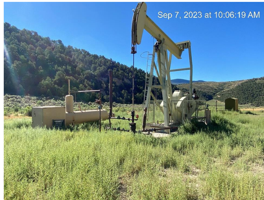
Pumping unit and separator
