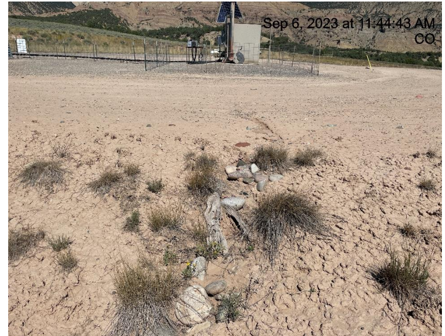
Photo # 8395 Check dams need maintenance
