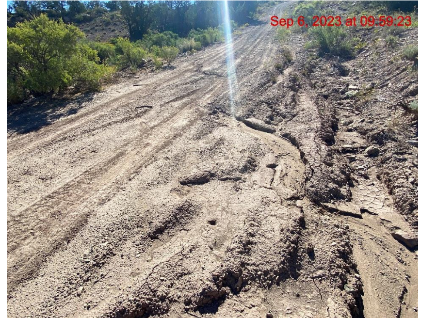
Access Road Erosion – Photo #06235
