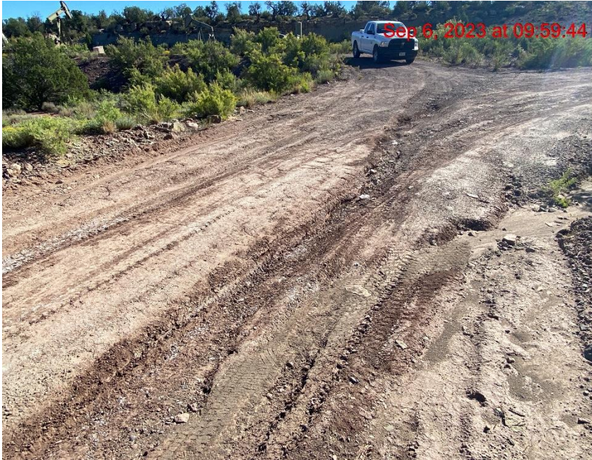
Access Road Erosion – Photo #06236
