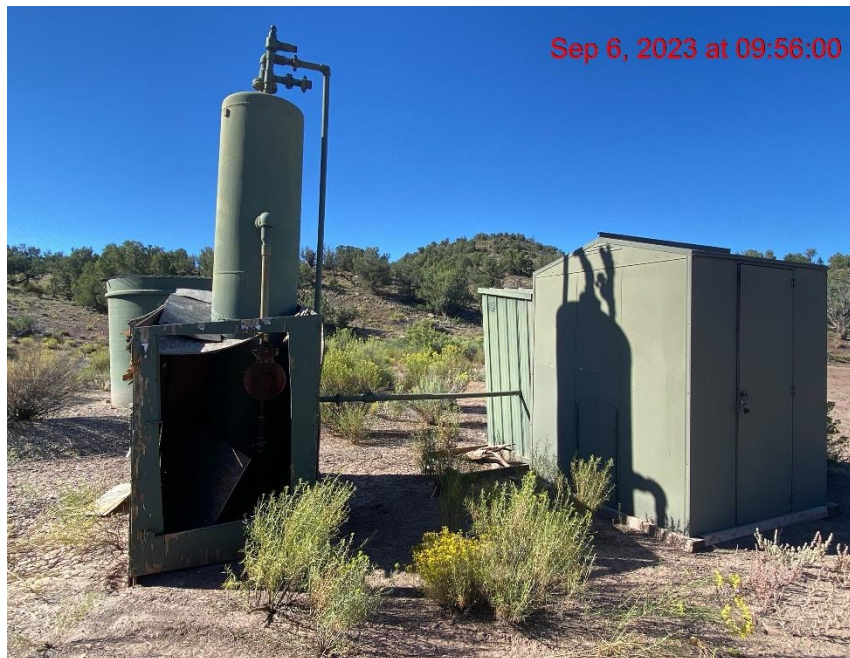
Separator/Gas Meter/Wildlife Entry Hazard/Weeds – Photo #06229
