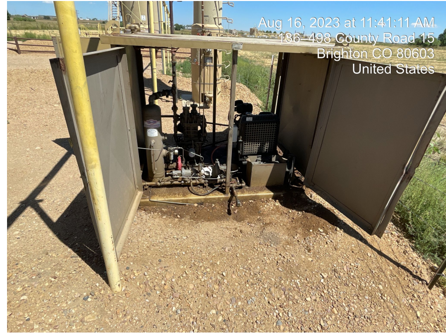
Photo 6. Photo of staining from leaking equipment on site facing west.
