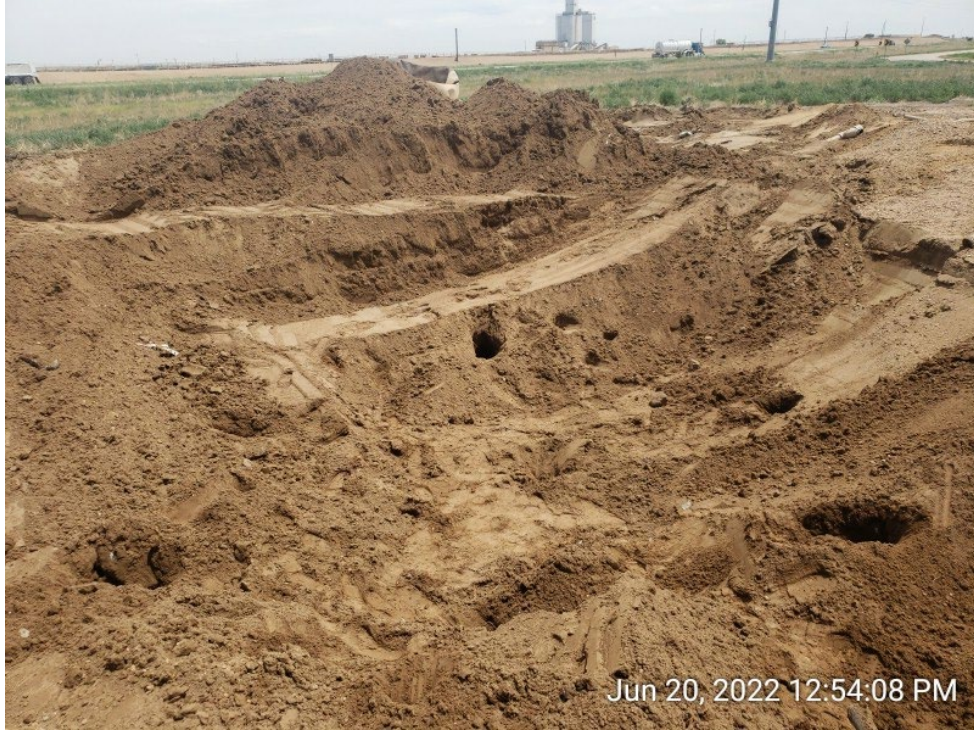
#4D - UPRC-65N64W 23SESW – Eastern Sidewall of Eastern Produced Water Vessel Excavation – EPWVE01@6.0' – No Impacts Noted – PID 0.8ppm – Facing East
