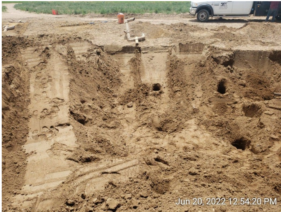
#4C - UPRC-65N64W 23SESW – Southern Sidewall of Eastern Produced Water Vessel Excavation – EPWVS01@6.0’ – No Impacts Noted – PID 0.6ppm – Facing South
