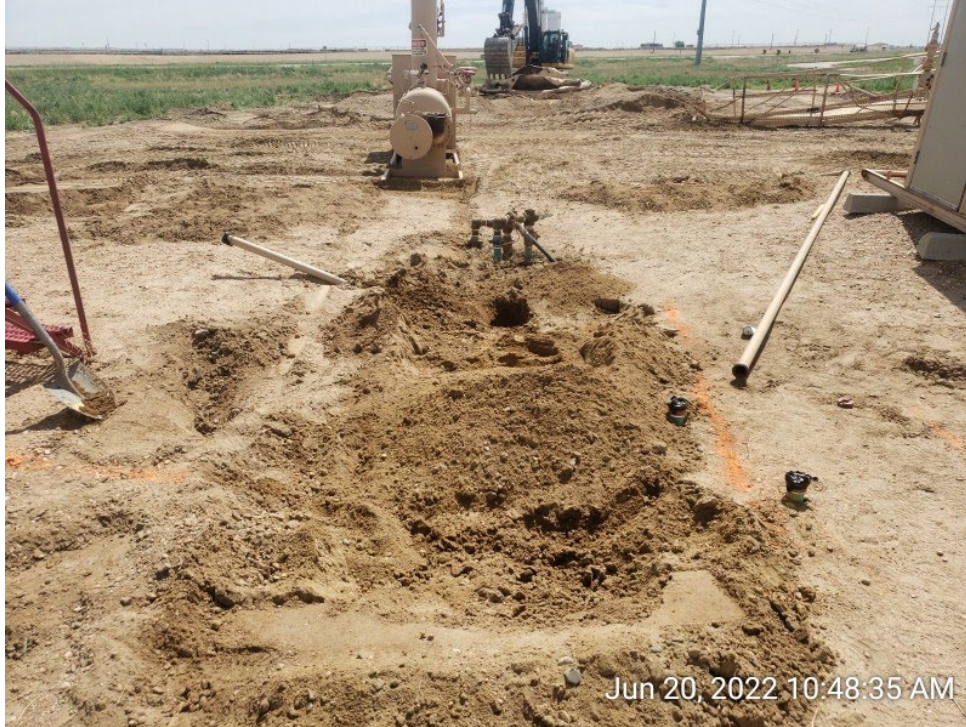
#7B - UPRC-65N64W 23SESW – Separator – SEP01@6.0” – No Impacts Noted – PID 0.3ppm – Sample Submitted for Lab Analysis – Facing East
