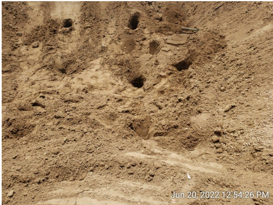
#5A - UPRC-65N64W 23SESW – Base of Western Produced Water Vessel Excavation – WPWVB01@7.0' – No Impacts Noted – PID 0.8ppm – Sample Submitted for Lab Analysis – Facing South
