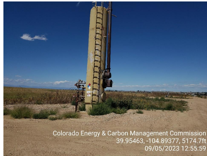
Photo 14 Heated Vertical Separator.
