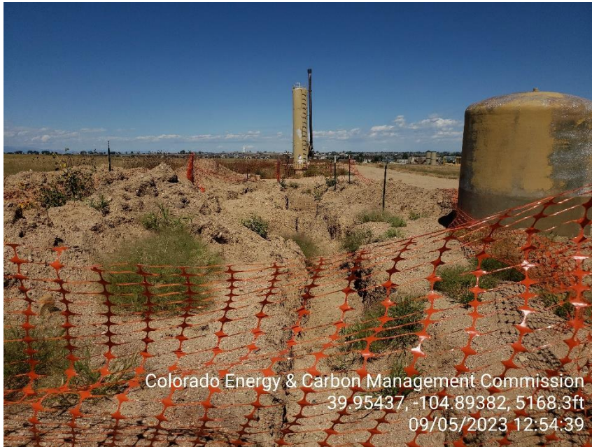
Photo 11 Flow line excavation.
