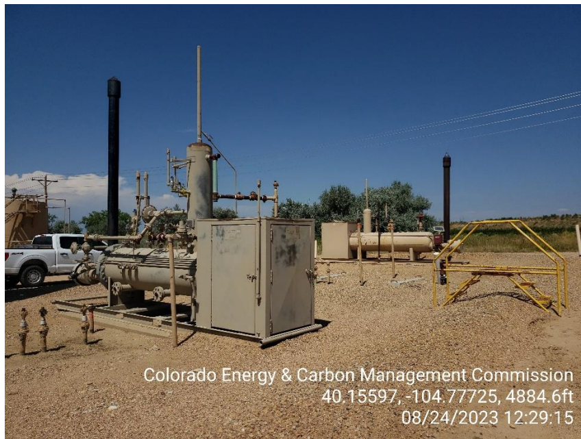
Photo 5 Horizontal Heated Separator.
