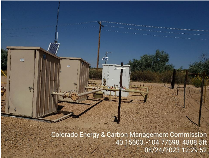
Photo 7 Gas Meter Run.
