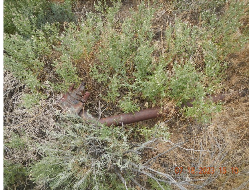
Flow line and valve daylighting in pit.
