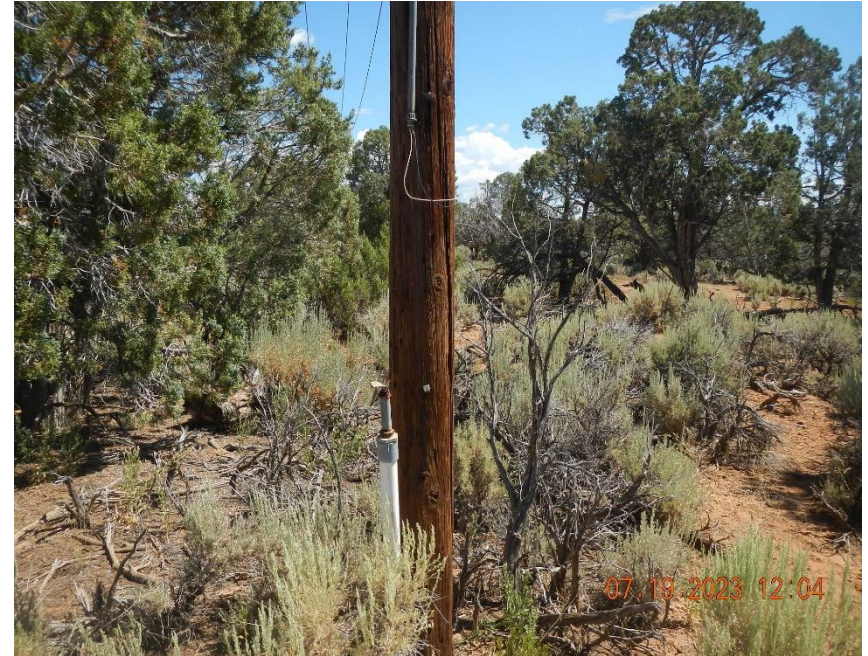
Electrical wires have been severed at the power pole.
