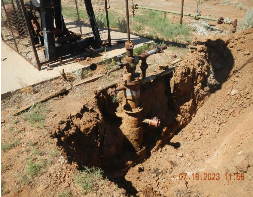
Open excavation around well head.
