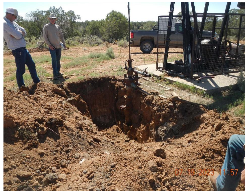
Open excavation around well head.
