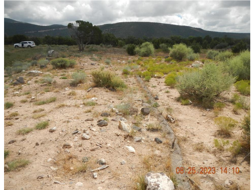
Wattles along southwest edge of location, along fill slope.
