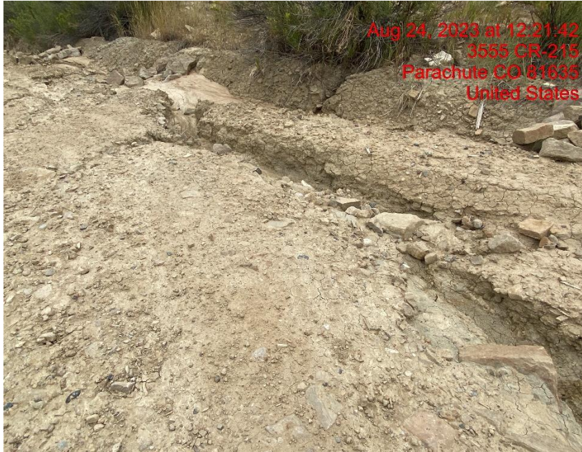
Insufficient Erosion Control/Rill Erosion on Access Road – Photo #06168
