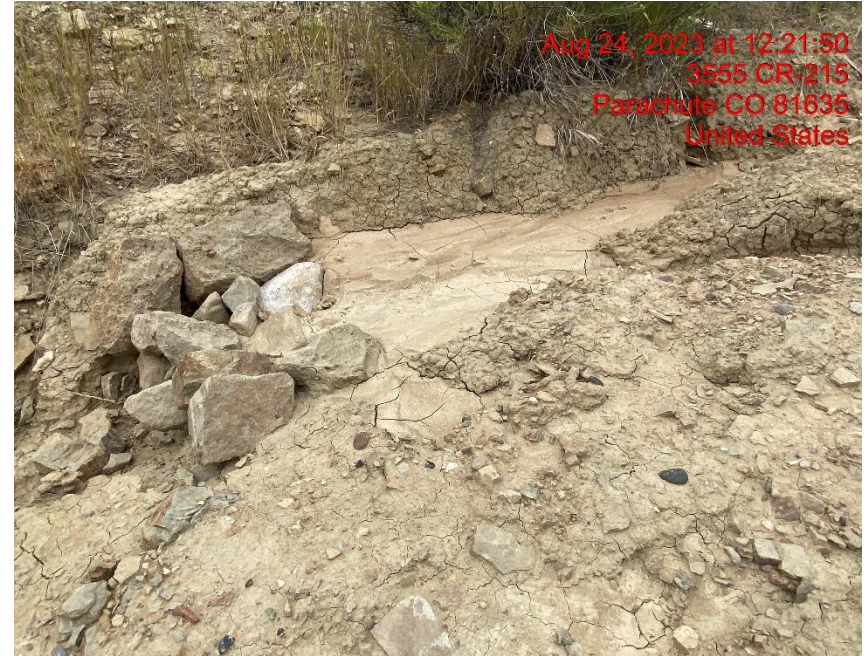
Check Dam BMP Needs Maintenance – Photo #06169
