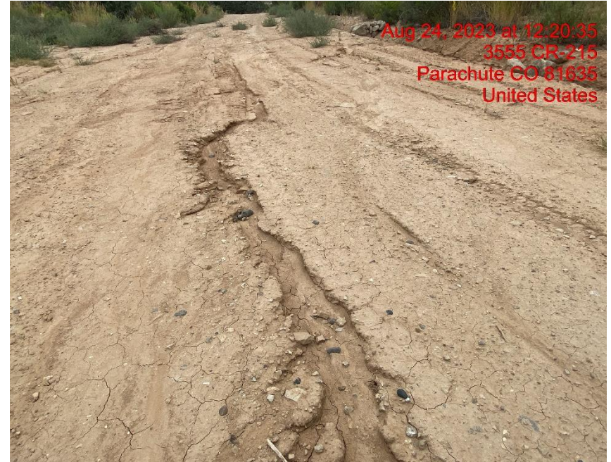
Insufficient Erosion Control/Rill Erosion on Access Road – Photo #06166
