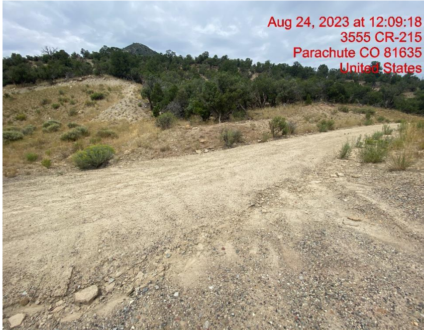
Insufficient Vehicle Tracking BMPs at Location Entrance/Exit – Photo #06163
