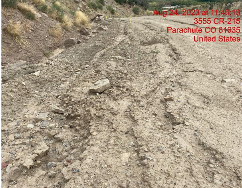
Access Road Degradation/Insufficient Erosion Control – Photo #06144
