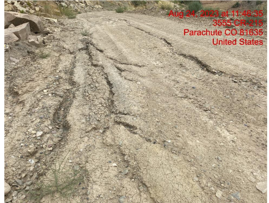
Insufficient Erosion Control/Rill Erosion – Photo #06146
