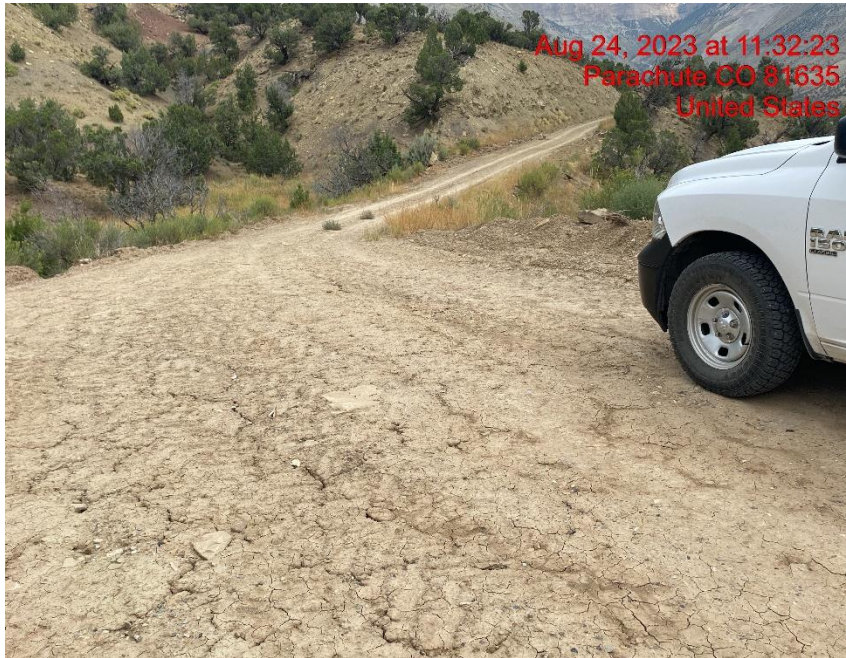
Insufficient Vehicle Tracking BMPs at Location Entrance/Exit – Photo #06141
