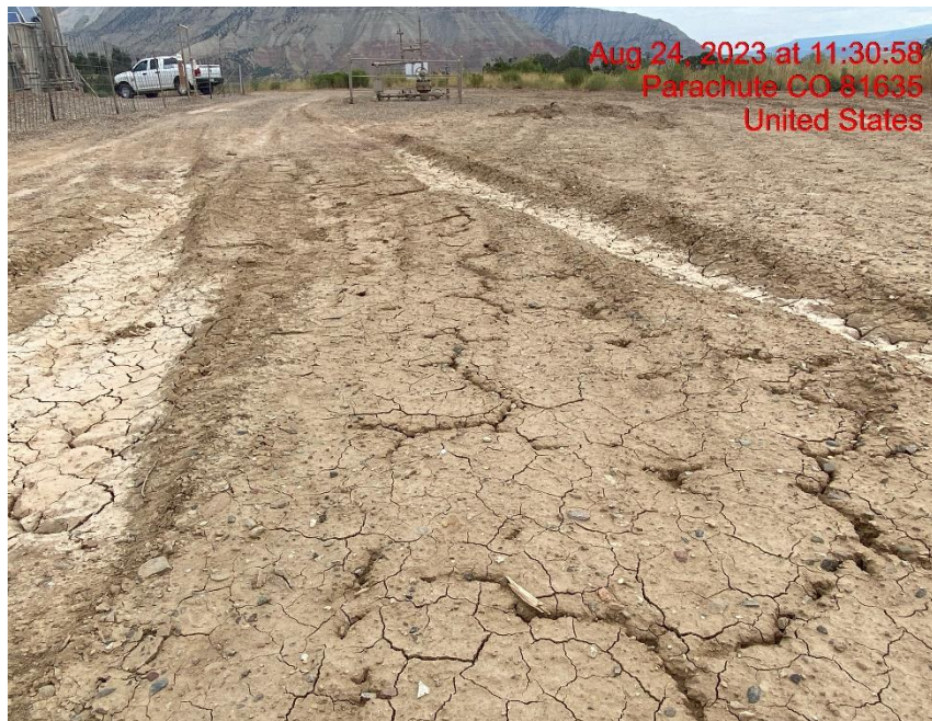
Location Lacks Stabilization – Photo #06134
