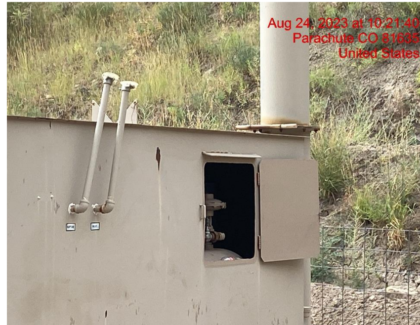
Unsecured Separator Hatch – Photo #06107
