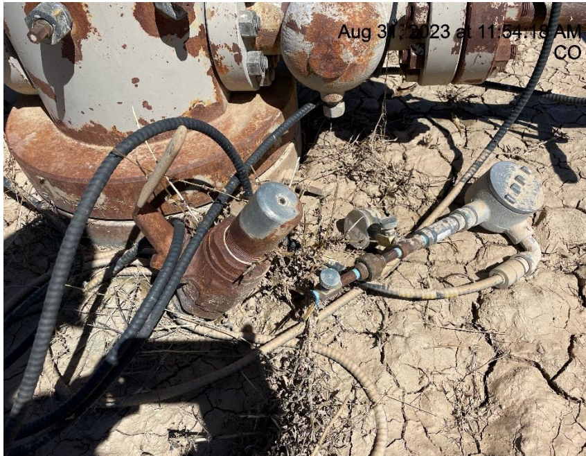
Photo # 7895 BENZEL 25-11 bradenhead line open to atmosphere
