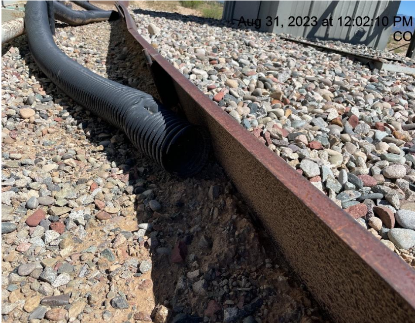
Photo # 7908 Flowline heating insulation open ended
