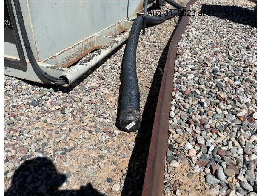
Photo # 7911 Flowline heating insulation no longer open ended, capped by Caerus employee. Please refer to equipment section of FIR for more information.
