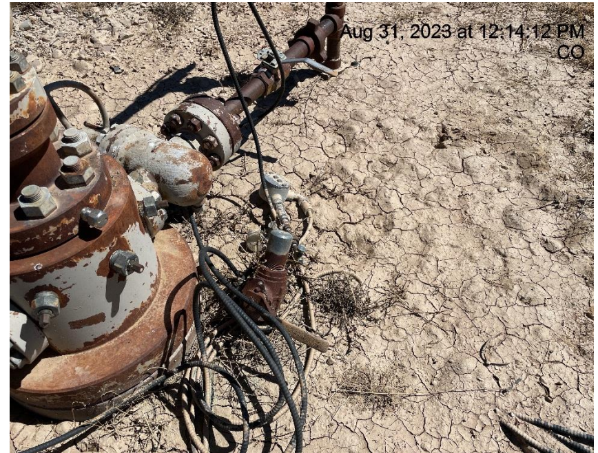
Photo # 7912 BENZEL 25-11 bradenhead line shut in at 2 inch ball valve by Caerus employee. Please refer to equipment section of FIR for more information.
