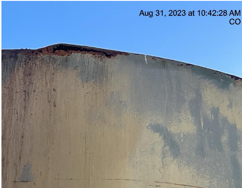
Photo # 7826 Hole in production tank/tank corrosion
