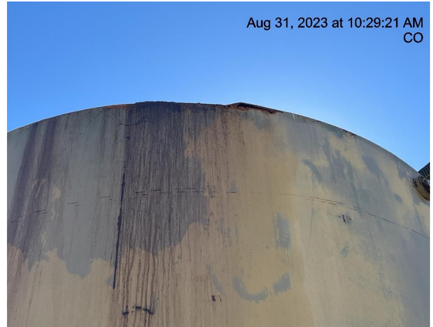
Photo # 7804 Hole in production tank/tank corrosion
