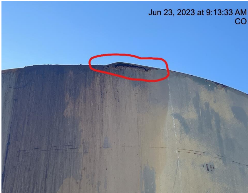
Photo # 1501 From inspection 708900837 conducted on 06/23/2023 Hole in production tank/tank corrosion
