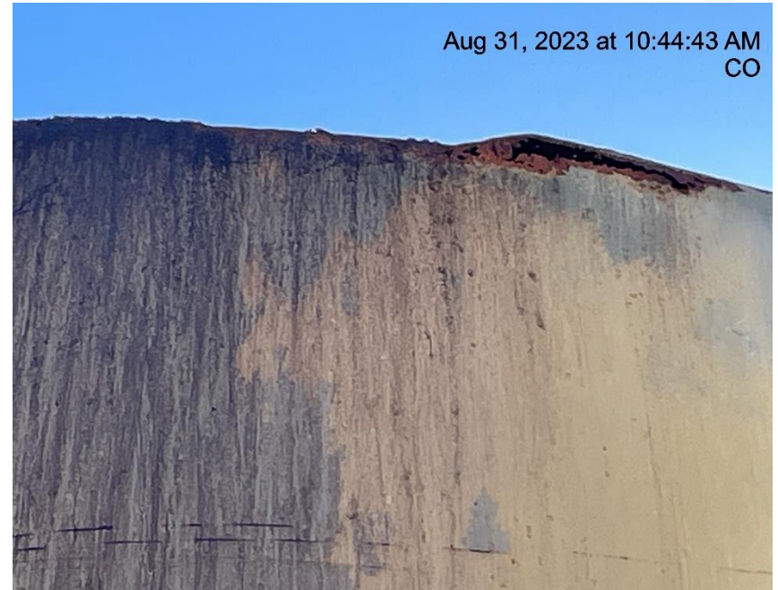
Photo # 7827 Hole in production tank/tank corrosion
