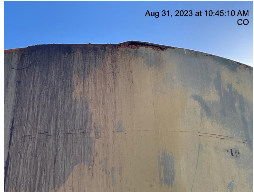
Photo # 7833 Hole in production tank/tank corrosion
